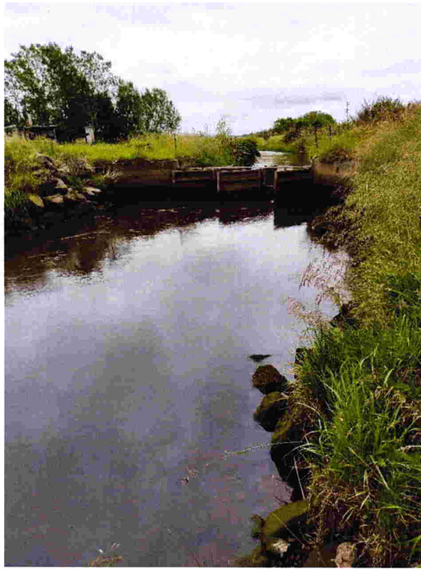
Photo 1: Titiroa Tide Gate Structure Opening, view upstream.
