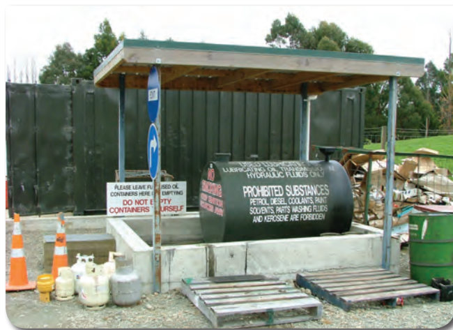
A bunded and covered area for storing used oil.
