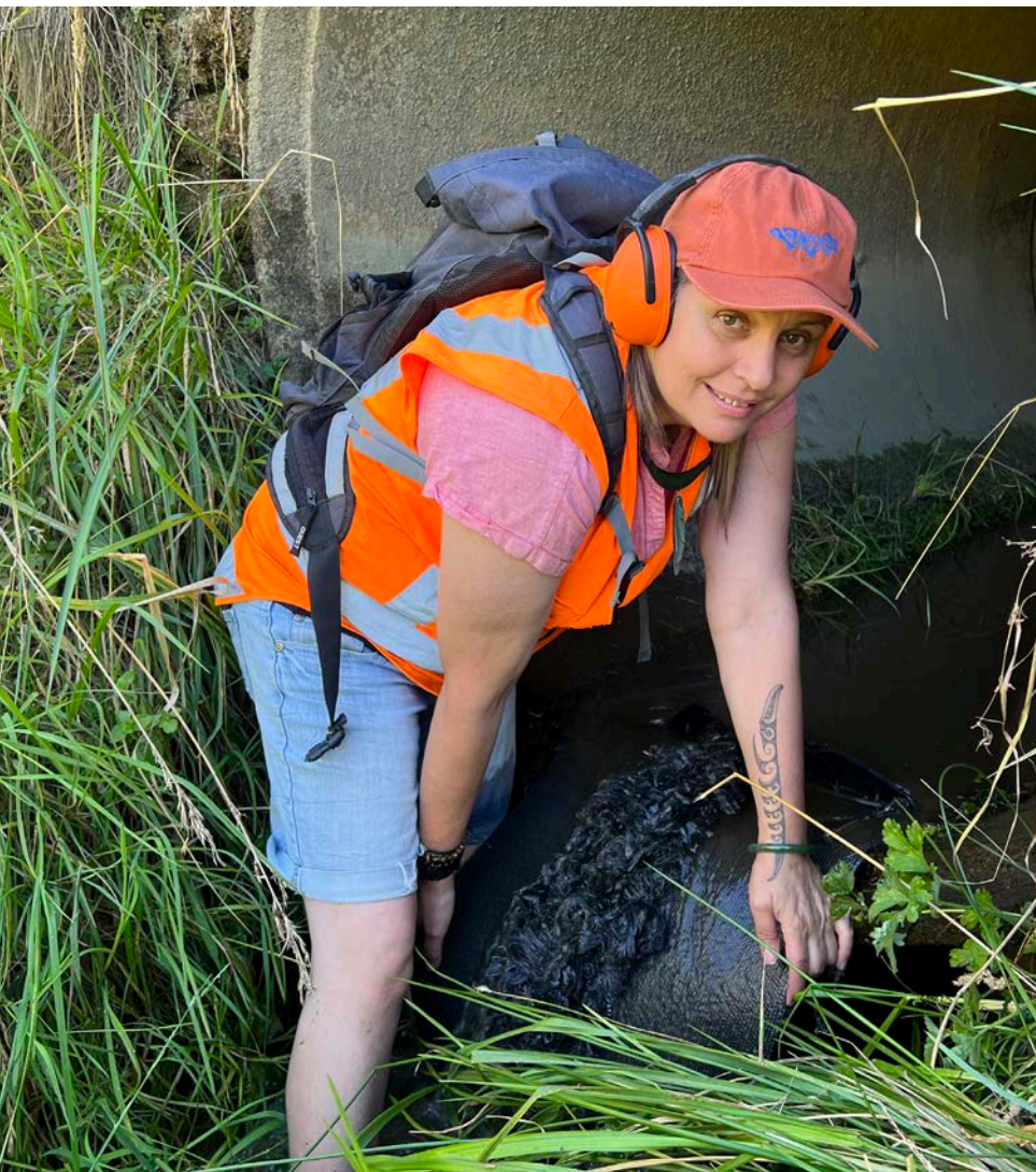
◀ Tania Kinita installing a rubber ramp and mussel rope.
