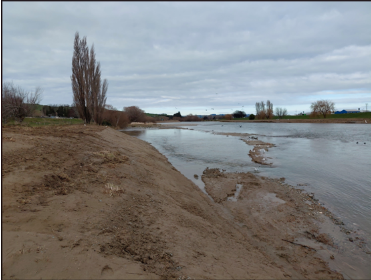
Photo2: Mataura Left Floodbank, Area 4, completed level – 28/7/26
