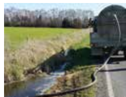
▶ A sucker truck should be used to remove effluent.
