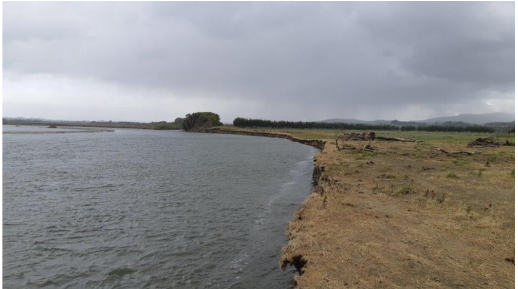
Figure 4 Bank erosion 2km downstream from Tuatapere - Jan 2020
