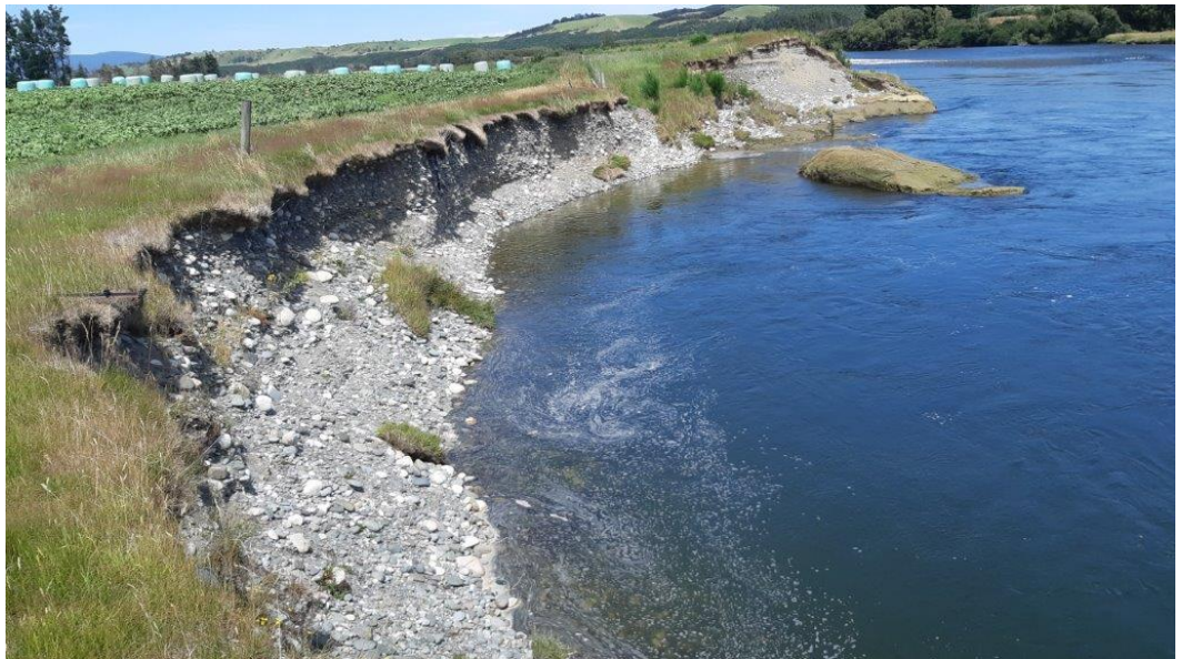
Figure 3 Bank Slumping 3kms upstream of Clifden - Jan 2020
