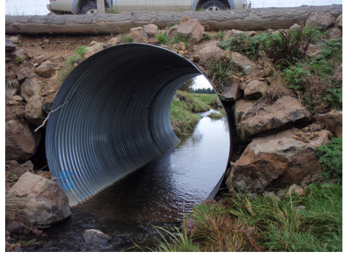
Good culvert placement, size and lane side baffles.
