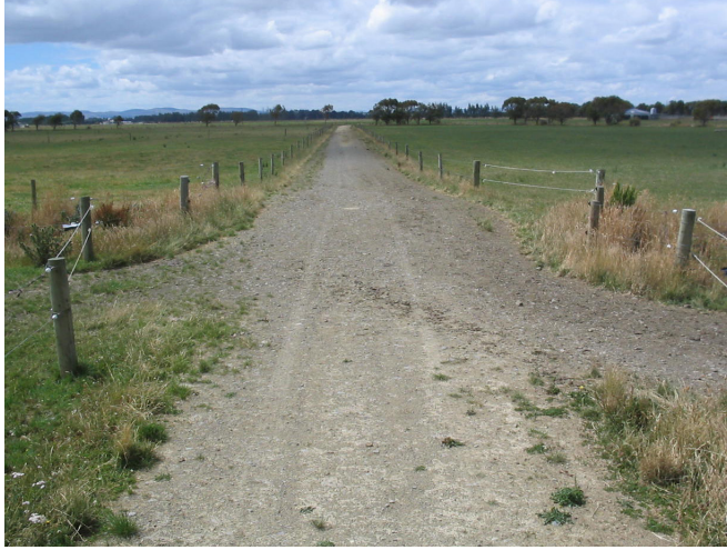
Good lane design with raised culvert, riparian strip and surface angles directing water onto pasture.
