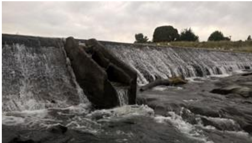
Figure 4. The Matura Weir summer 2017. Note salmonid ladder at centre weir. Photo courtesy Alliance. (from Vaipuhi 2018b)
