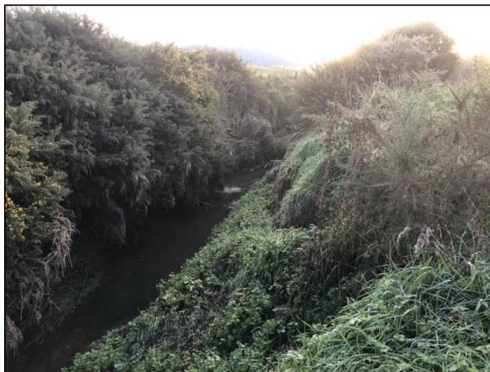
Photo 7: Proposed Sediment Trap Location – East Side and South of Pine Tree Plantation
