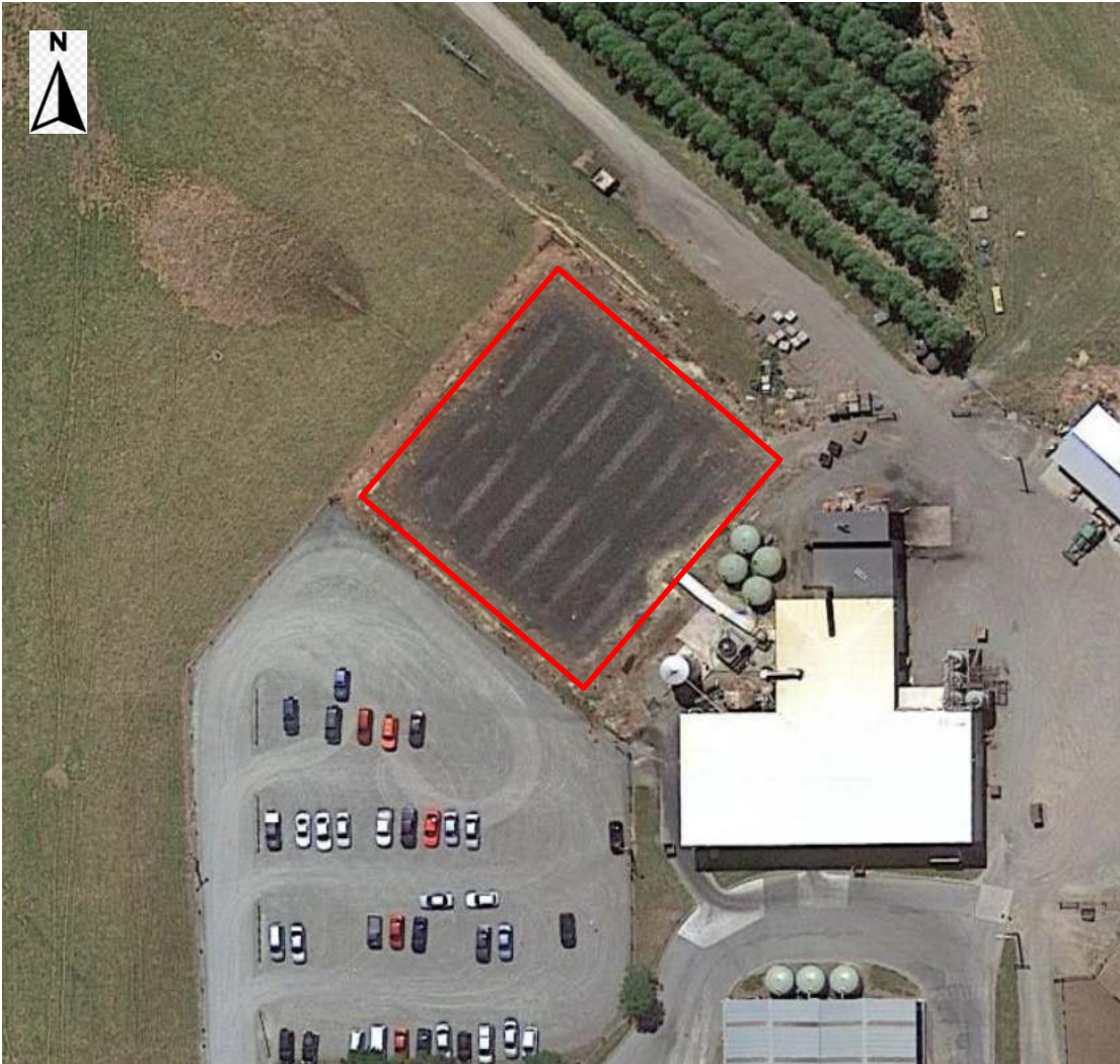
Figure 1. Biofilter Location (within the red rectangle)
