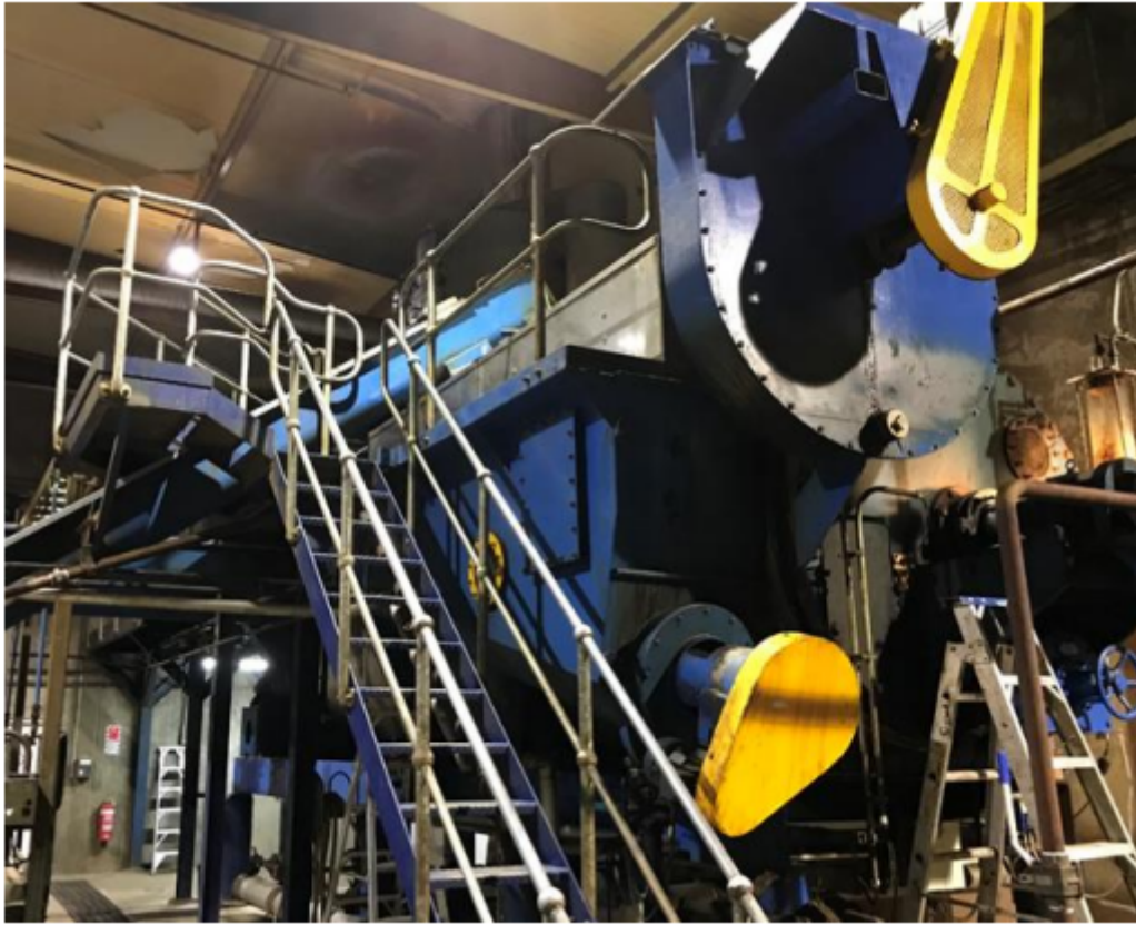
Figure 4 Continuous cooker in rendering plant
