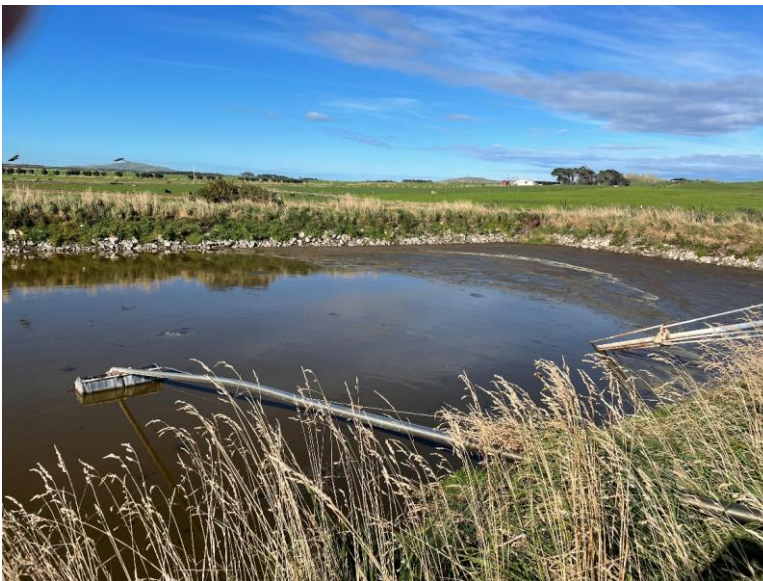
Main Effluent Pond showing vegetative buffers
