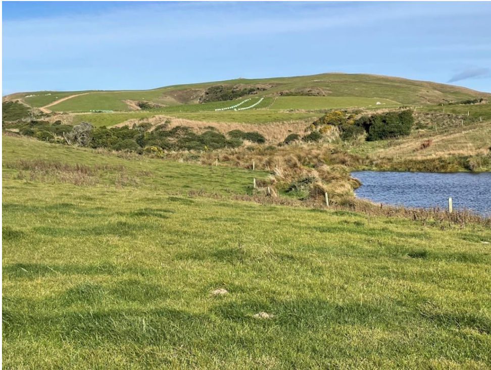
Fenced dam and vegetative buffers, fenced bush and riparian filter prior to dam
