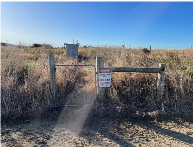
Fencing around effluent pond showing vegetative buffer and signage
