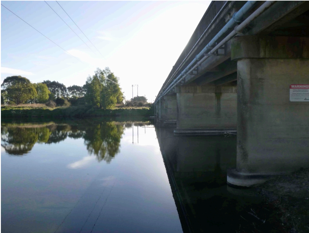
Figure 2. Wyndham and Edendale wastewater treatment system discharge ‘droppers’ on the southern side of the Edendale-Wyndham Road bridge, April 2021.
