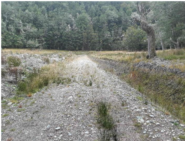
View west along east-west track. Northern side of track cuts into wetland, but track cuts less into substrate on south side.
