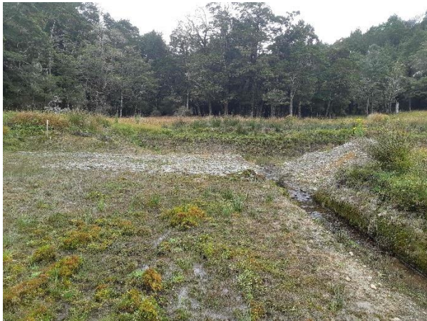
View north across Red area. Area in foreground has been stripped back to clay. Upper centre shows that excavation has intercepted wetland.
