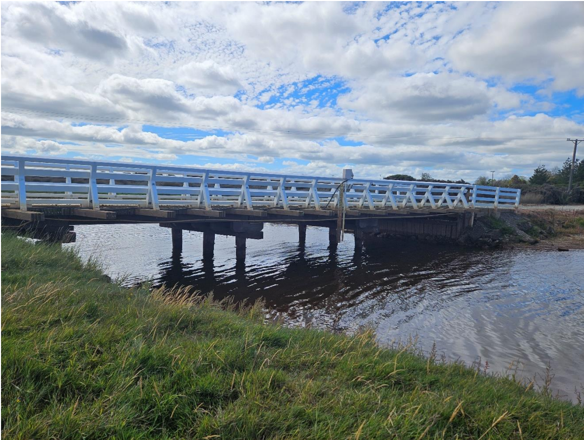
Figure 6: Waghorn Road Bridge, looking upstream and showing gauge location on the bridge
