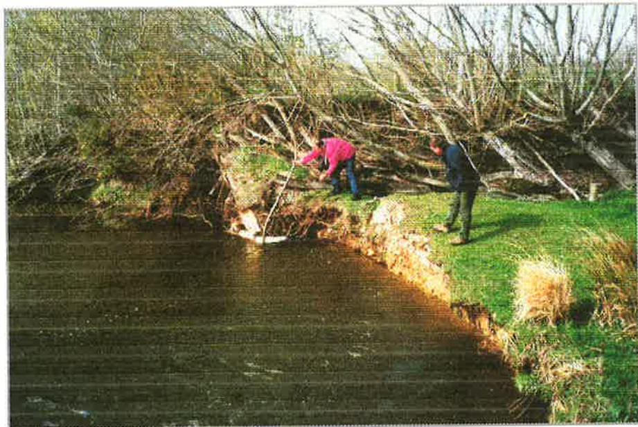
Figure 6. Unchannelized reach upstream. The deepest observed scour hole was ~1 m at low flow.
