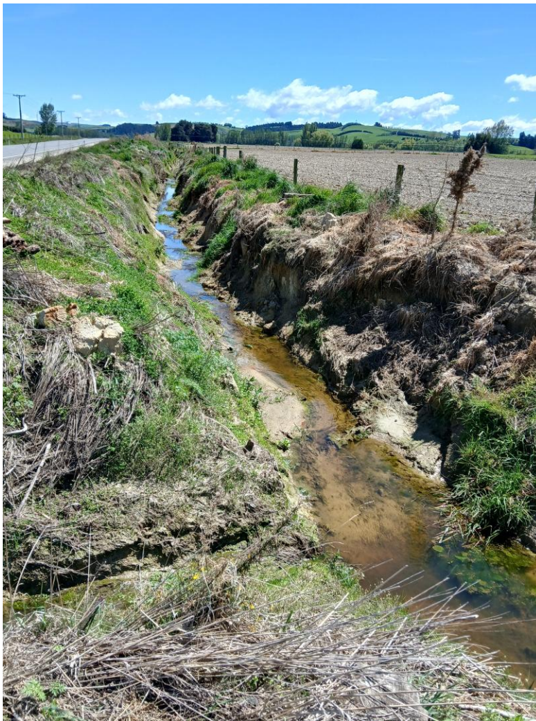
Figure 2- Western drain, upstream of the proposed site, post drain clearing.
