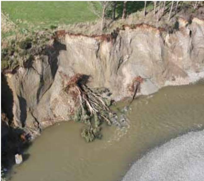
River bank erosion
