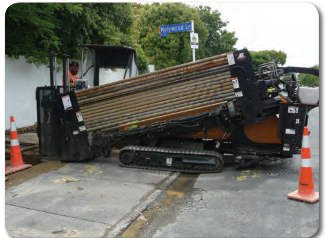
A directional drill at work.
