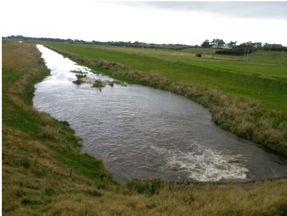
Figure 1.2: The Waihopai Dam, view downstream
