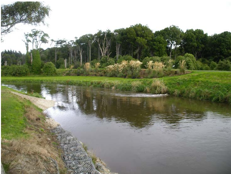
Figure 2.1: Waihopai River, downstream of Queen's Drive Bridge
