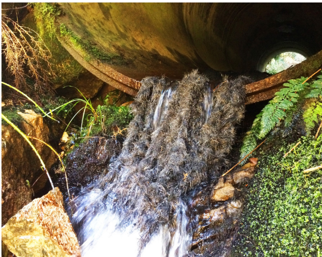
▶ Mussel rope can be installed to help climbing species make their way up into and on through culverts. (Photo: ATS Environmental)
