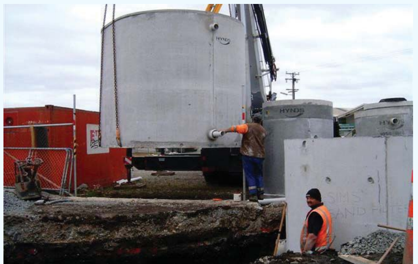
A stormwater treatment system was installed on the site as part of the clean up.
