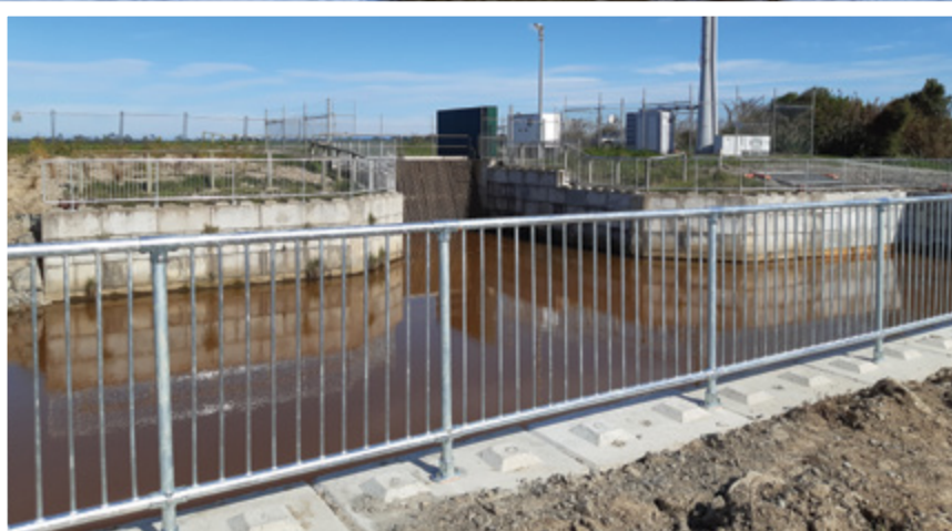
▲ The new sediment pond near the bottom of Beatrice Street (above and background).
