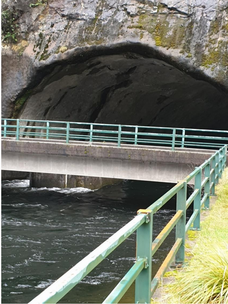
Figure 4: The waters of the Waiiau River exiting a discharge tunnel at Deep Cove in Doubtful Sound (source: WRG Submission on the NPSFM 2020).
