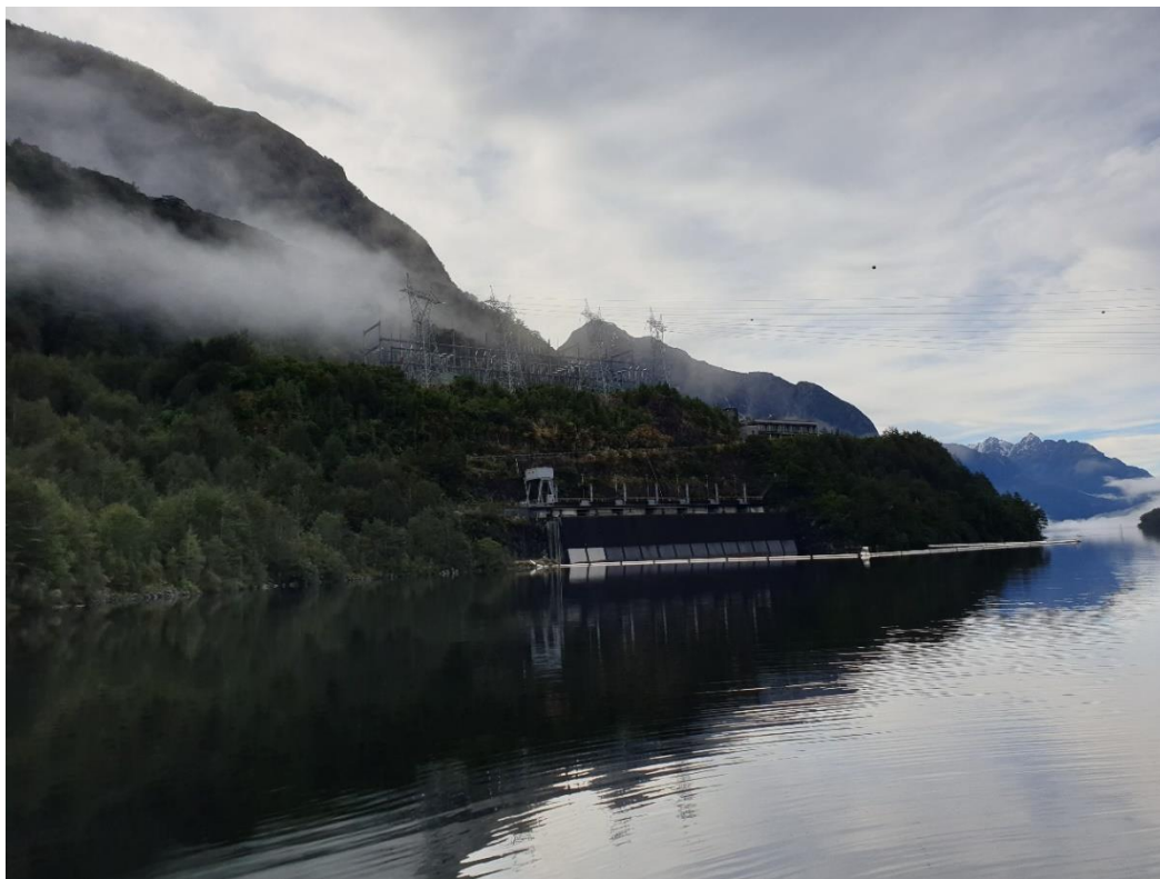
Figure 5: The Manapouri Power Station at West Arm, Lake Manapouri (source: WRG Submission on the NPSFM 2020).
