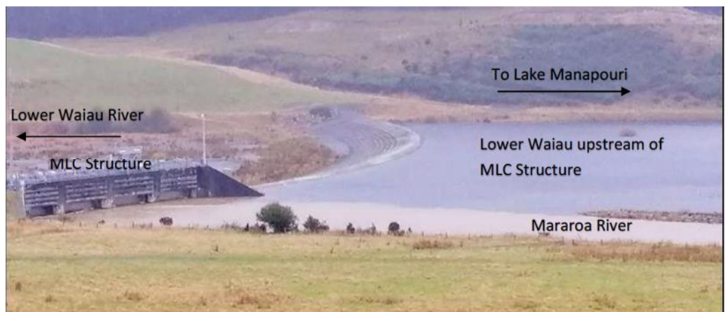
Figure 3: The Manapouri Lake Control Structure diverting sedimented Mararoa waters through the Weir to the lower Waiiau River (source: WRG Submission on the NPSFM 2020).
