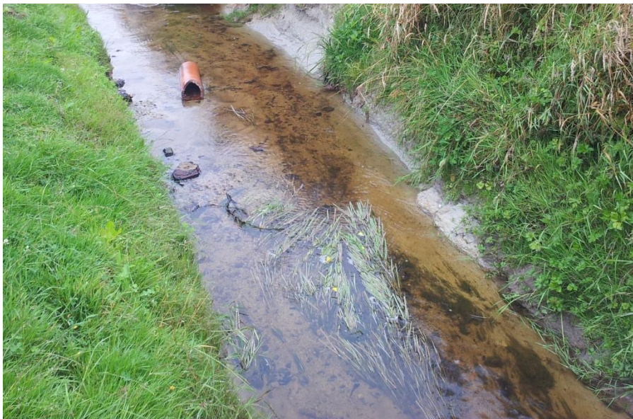
Figure 5: In stream cover for fish and invertebrates is usually removed by drain clearing.
