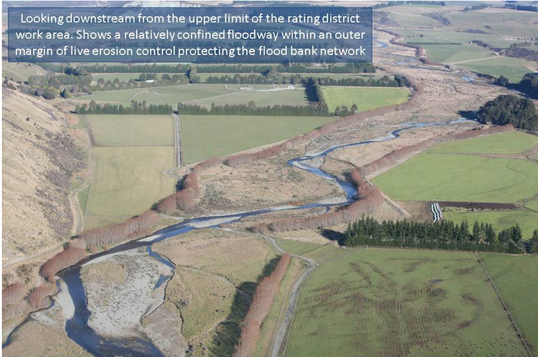
Draft Concept Plan – River Corridor Vegetation Management Image 5 – Upper Whitestone River - (D0561 #1580)
