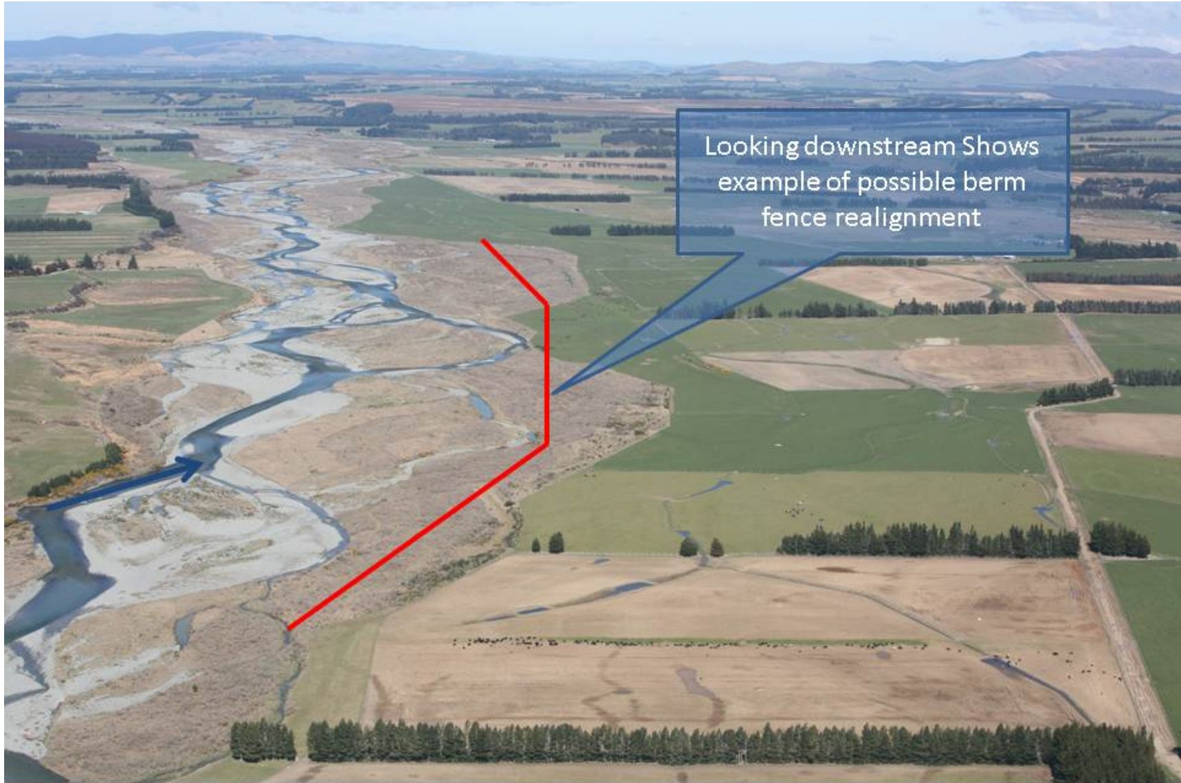
Draft Concept Plan – River Corridor Vegetation Management Image 1 – Upper Oreti River (D0552 #8200)
