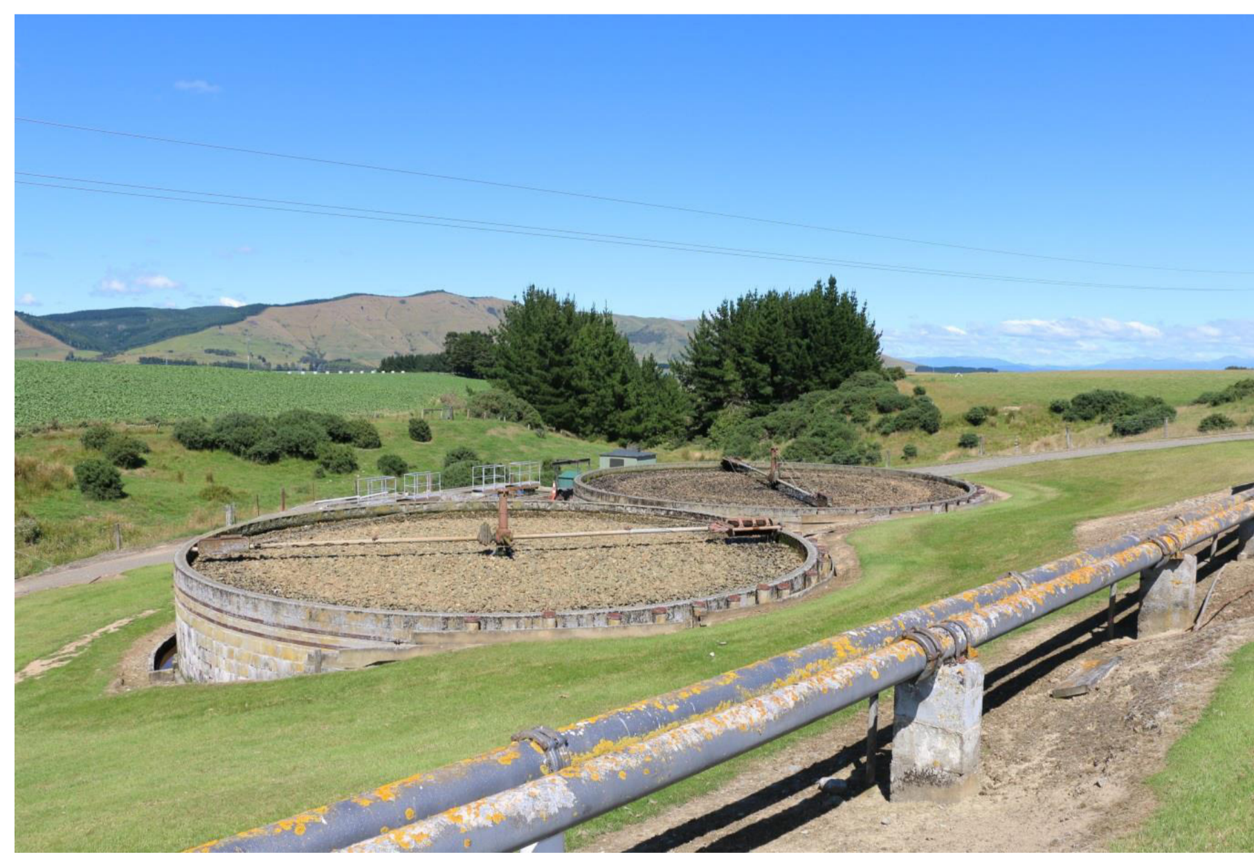
▲ Ohai biological trickling filter with tributary of Orauea Stream between pine trees
