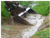
Surface drain maintenance
