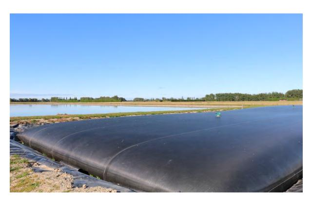
Image C6: Winton desludging geobag with oxidation pond in background
