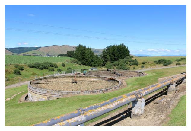
Image C8: Ohai biological trickling filter with tributary of Orauea Stream between pine trees
