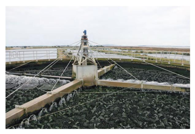
Image C16: Clifton wastewater trickling filter
