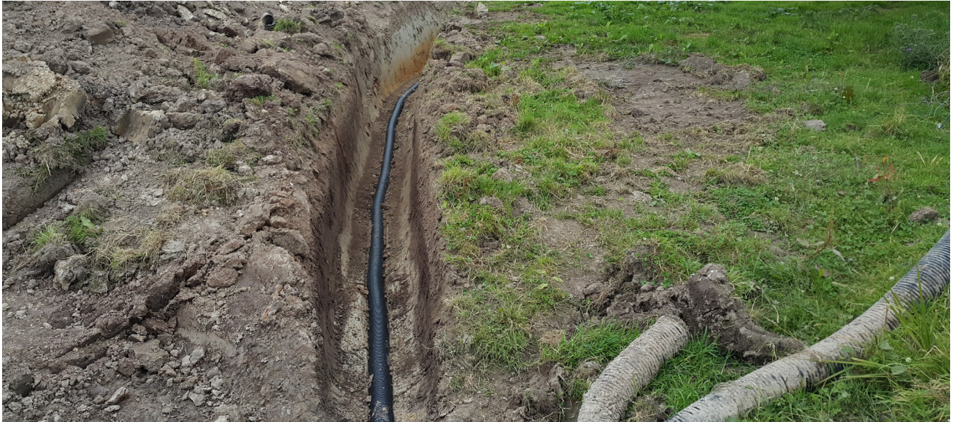
New tile drain
