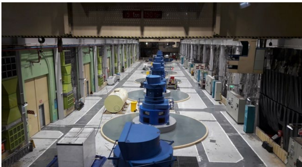
Figure 10: Turbine Hall - Manapouri Power Station
