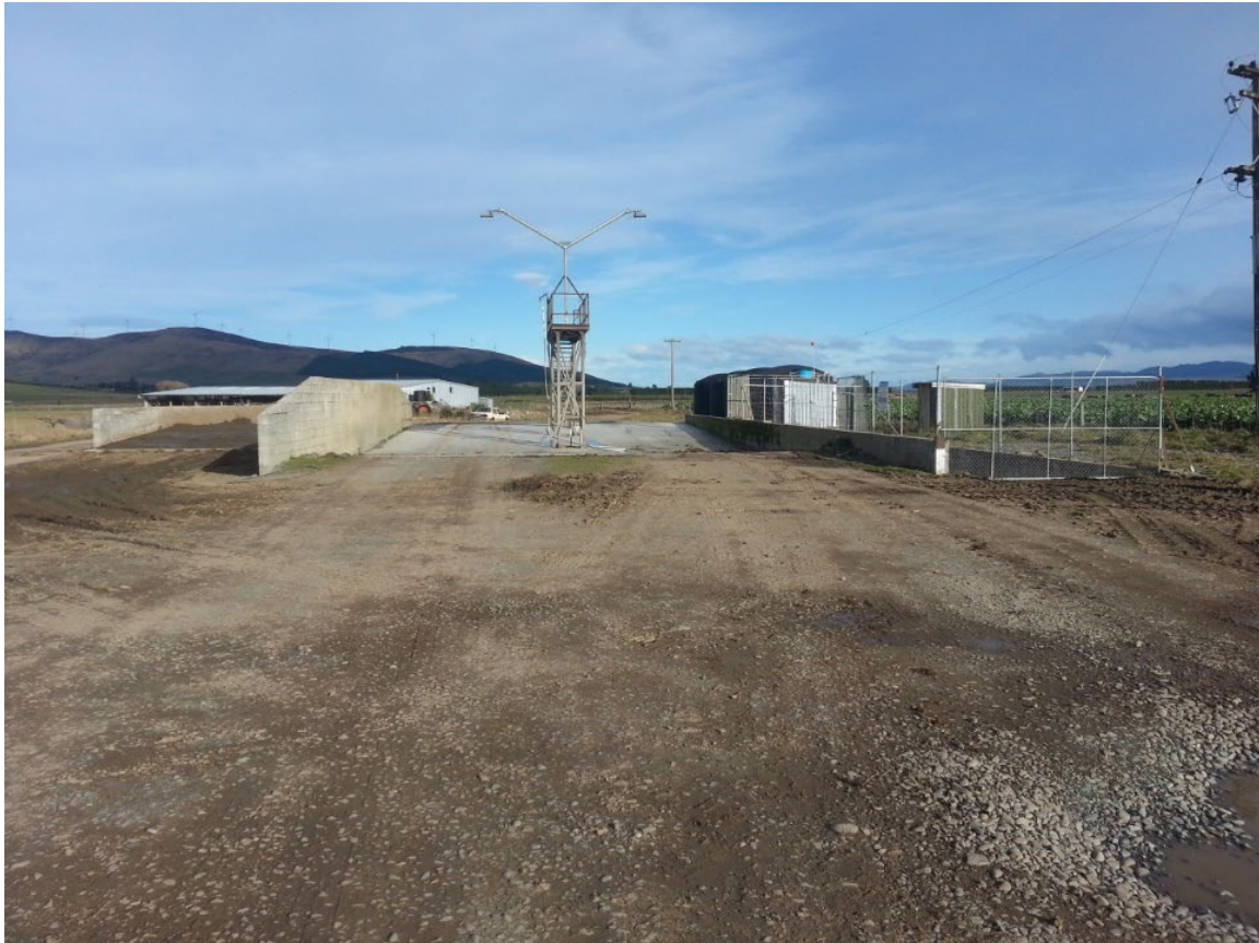
Figure 23: An example of a truck wash facility
