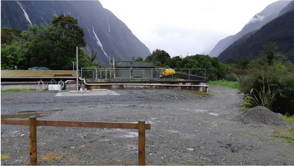
Figure 21: Milford Sound wastewater treatment plant
