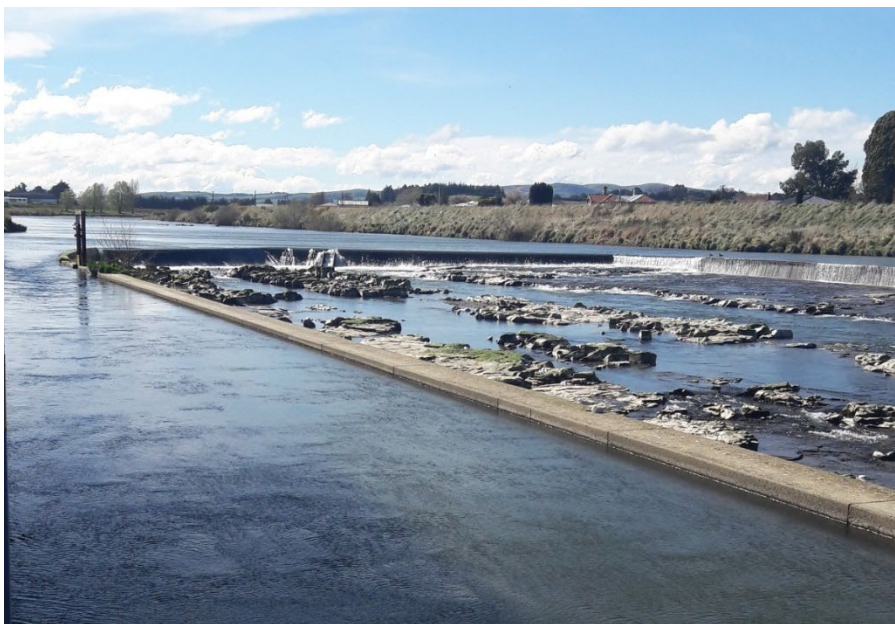
Figure 7: Upstream sampling site, Alliance Group Mataura Plant
