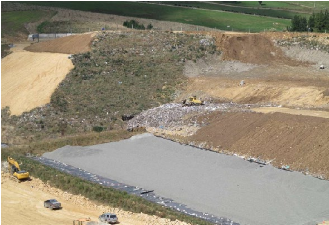
Figure 17: View of active filling in area 15 with area 14 behind, AB Lime
