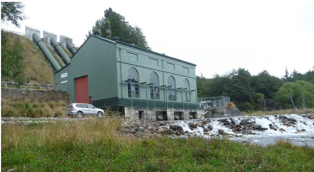
Figure 9: Monowai Power Station
