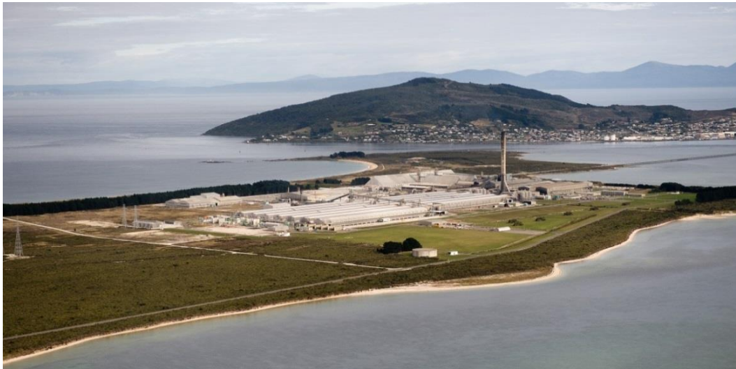
Figure 14: Aerial view of NZAS site. (Image by NZAS)
