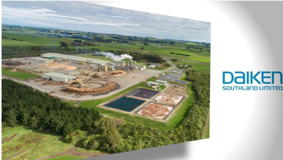
Figure 15: Aerial view of Daiken Southland site (Image by Daiken Southland Limited)
