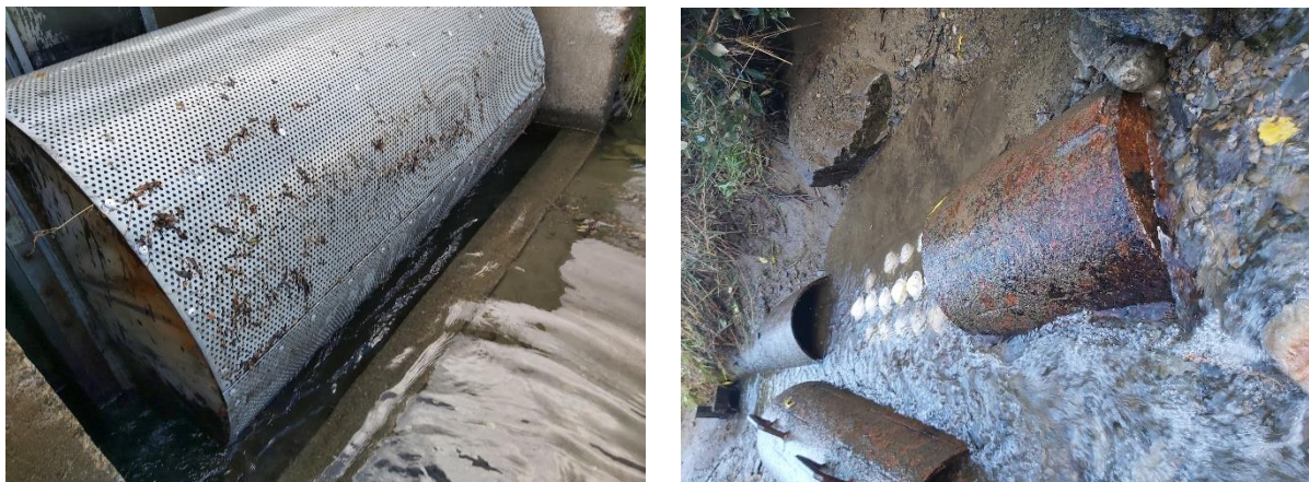
Figure 8: An example of a rotating drum screen and of another fish screen design
