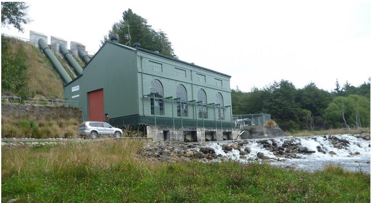
Figure 12: Monowai Power Station
