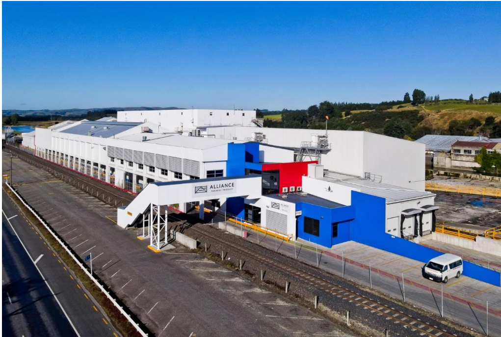
Figure 10: Alliance Maitai Plant
