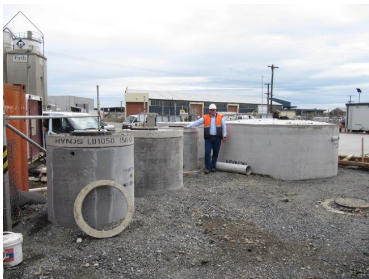
Figure 77: Stormwater treatment system prior to installation, February 2011 (photo supplied by Sims Pacific Metals).
