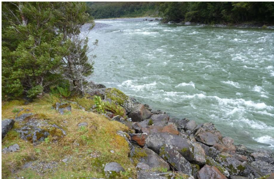
Figure 66: Existing rip rap river bank protection behind Milford Lodge, March 2011.
