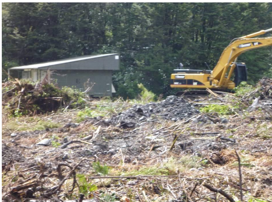
Figure 64: Clearance of Cleddau Village platform, March 2011.
