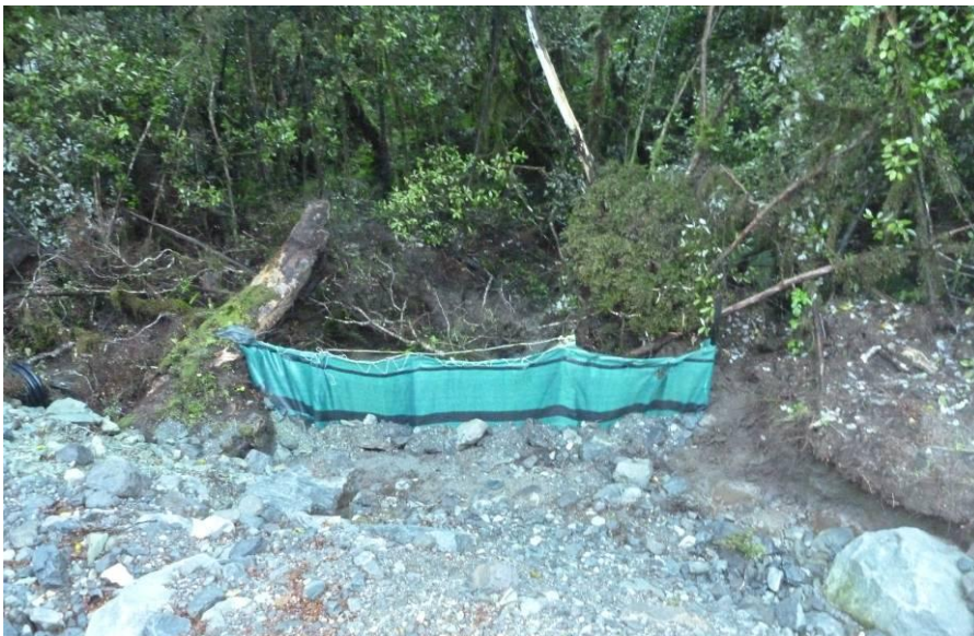
Figure 69: Sediment control at borrow area, 15 June 2011.
