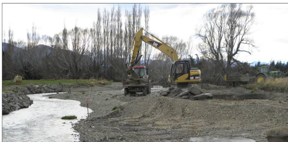
Figure 51: Gravel Extraction to construct a sediment trap on the Hamilton Burn.
