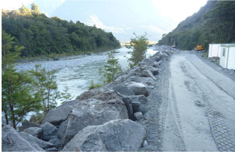
Figure 70: Newly constructed rip rap flood wall behind Milford Lodge, 15 June 2011.
