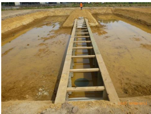
Figure 27 - An example of the construction of additional effluent storage similar to that required by the two recent enforcement orders
