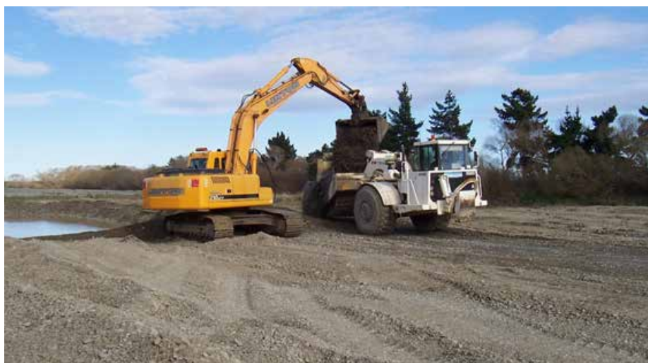
Figure 15 - Gravel extraction, Oreti River, upstream of the Winton Bridge
