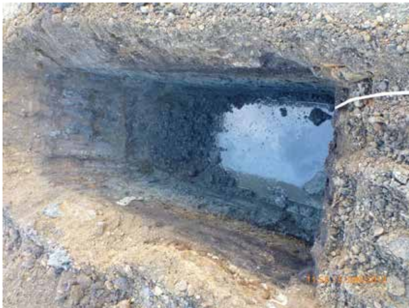
Figure 31 Excavated hole showing extent of contamination
