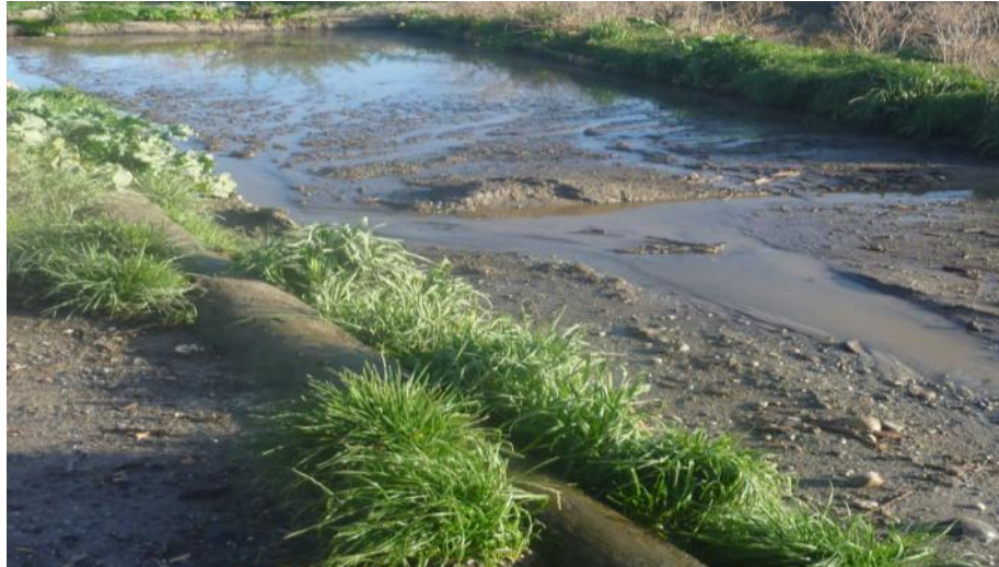
Figure 20 - Sealed runoff area to capture sediment from truck wash
