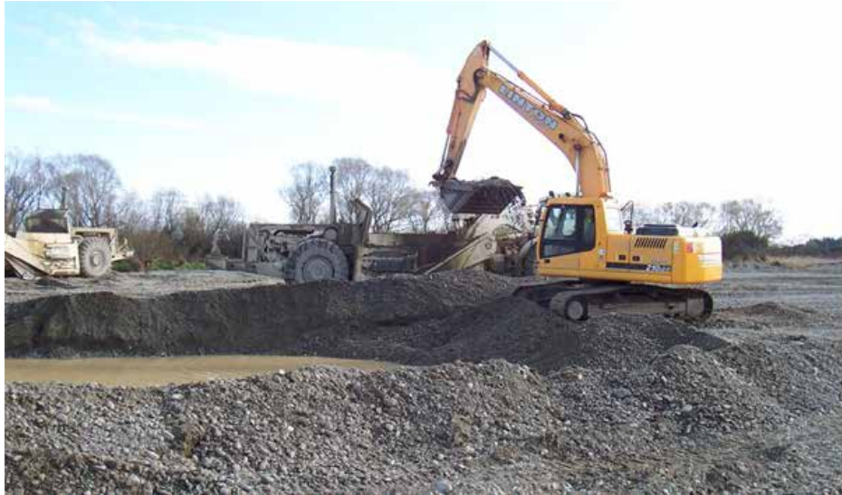
Figure 16 - Gravel extraction, Oreti River upstream of the Winton Bridge
