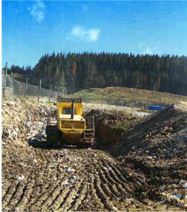
Landfill compactor in action
