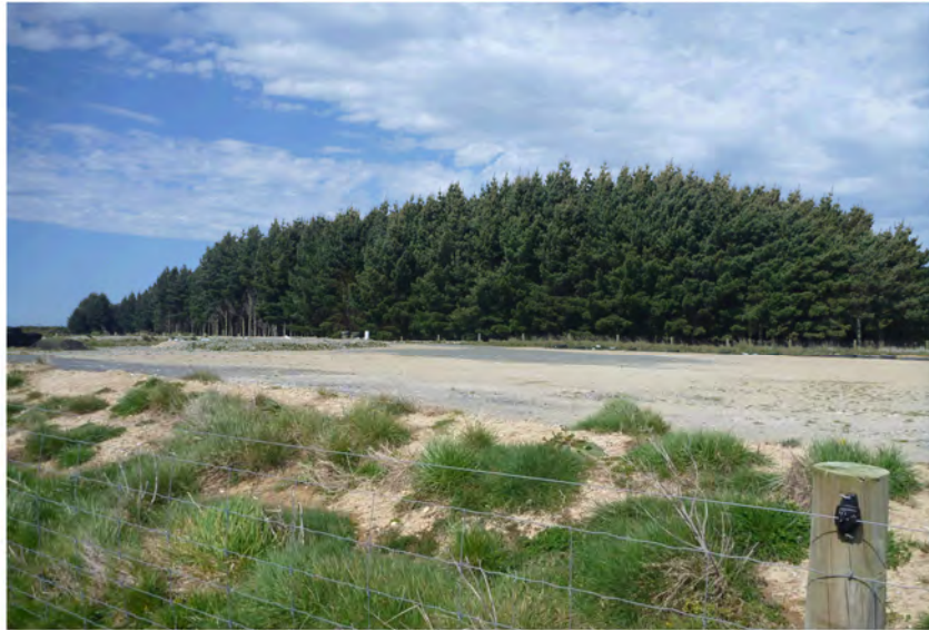
Holding pad for retaining contaminated soils for sampling and encapsulation of contaminants.
