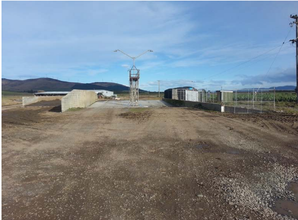
Example of good practice at Northern Southland Transport's truck wash.
