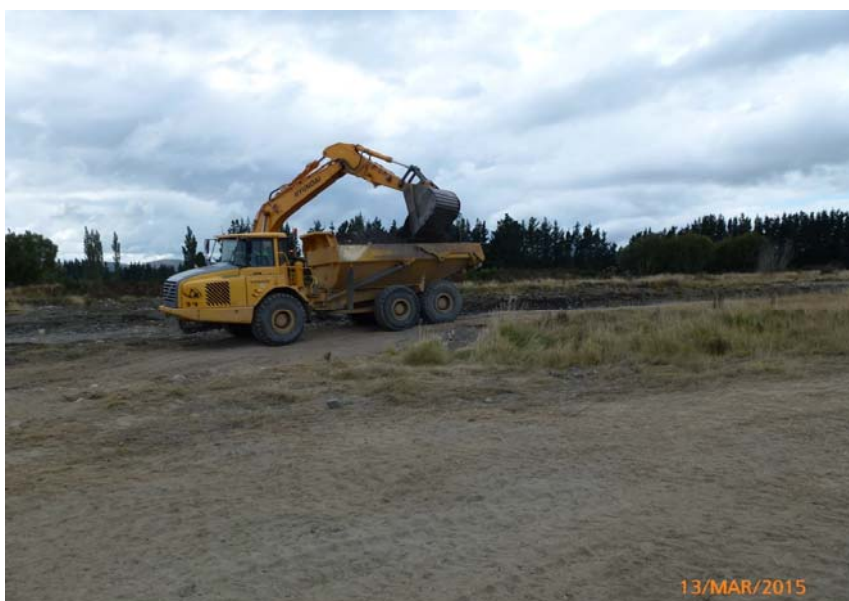
Aparima River at Jacobs Bridge, new channel excavation and gravel extraction
