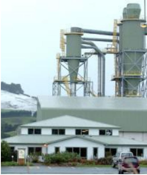
Dongwha site office.
