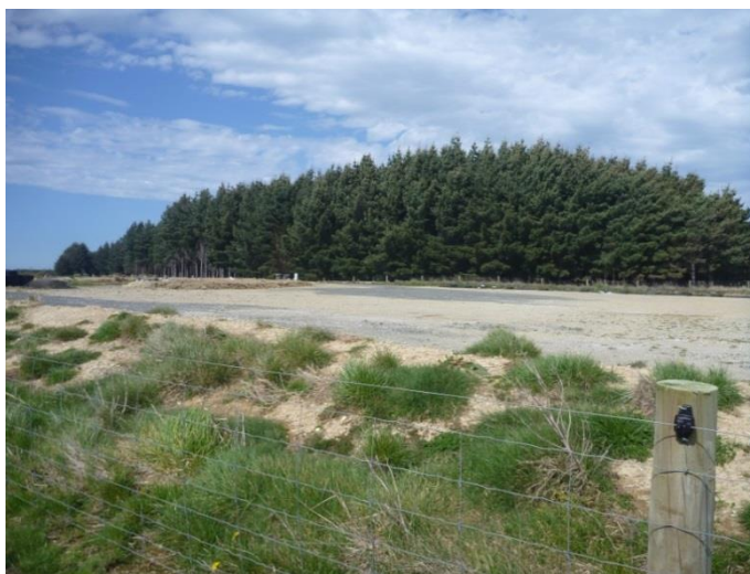
Holding pad for retaining contaminated soils for sampling and encapsulation of contaminants.
