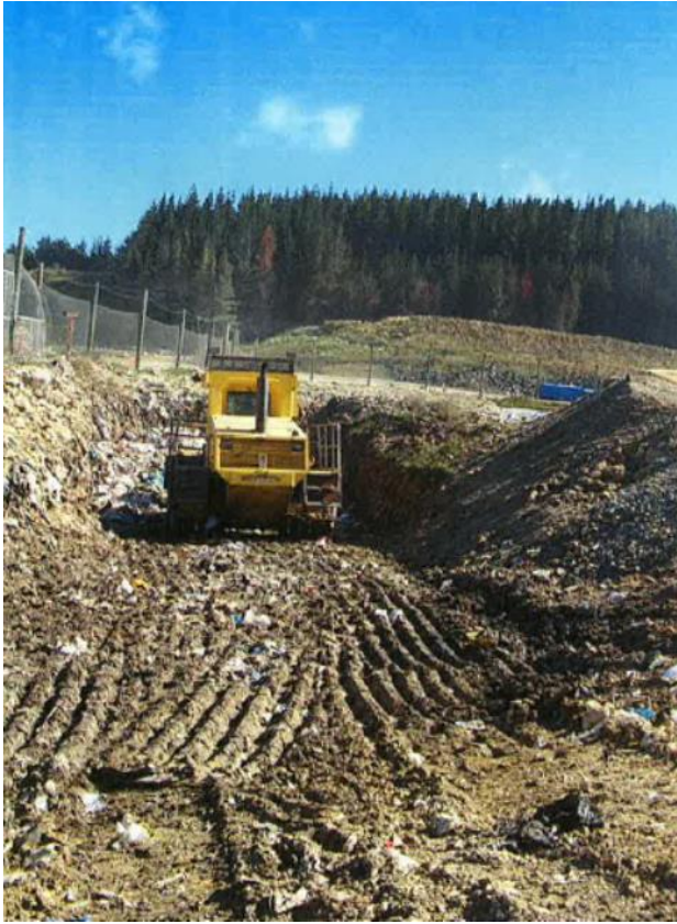
Compactor in action.
