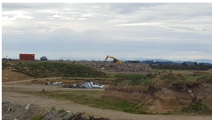
Cleanfill and limited scope landfill site.
