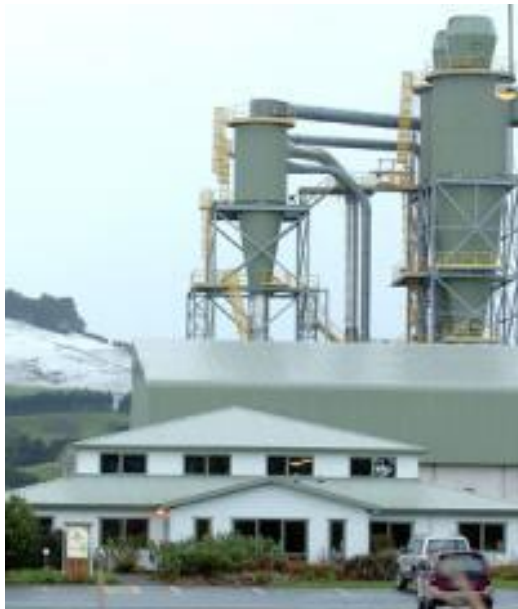
Dongwha site office.
