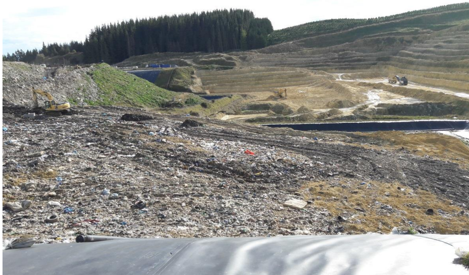
View across areas 13 and 14 of the active landfill, AB Lime
