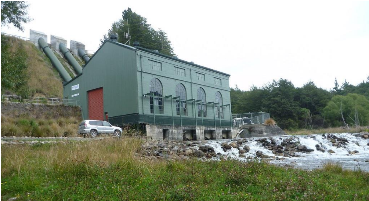
Figure 9: Monowai Power Station
