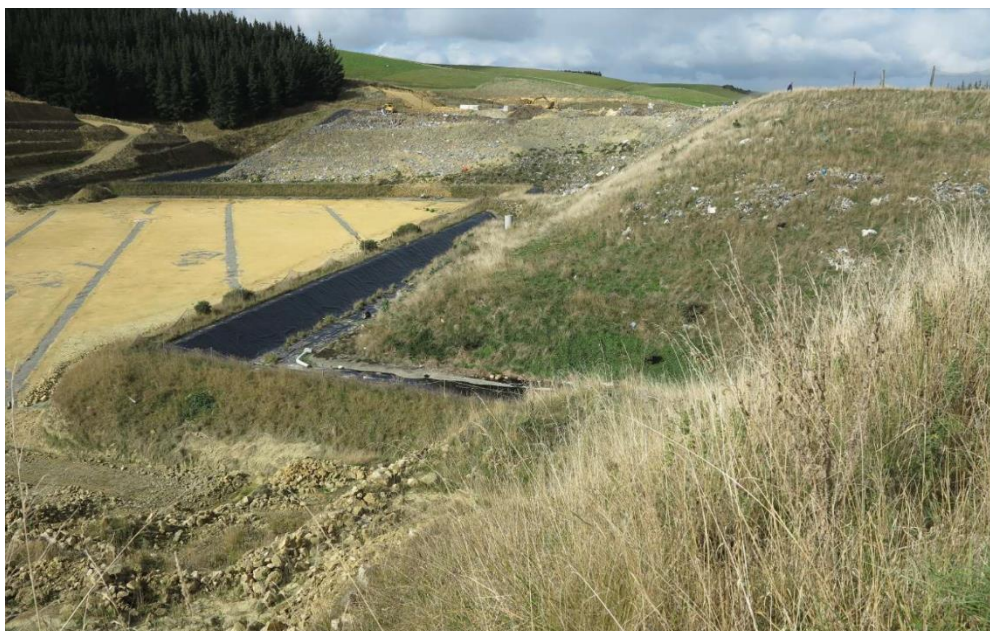
Figure 17: View across areas 14 of the active landfill, AB Lime
