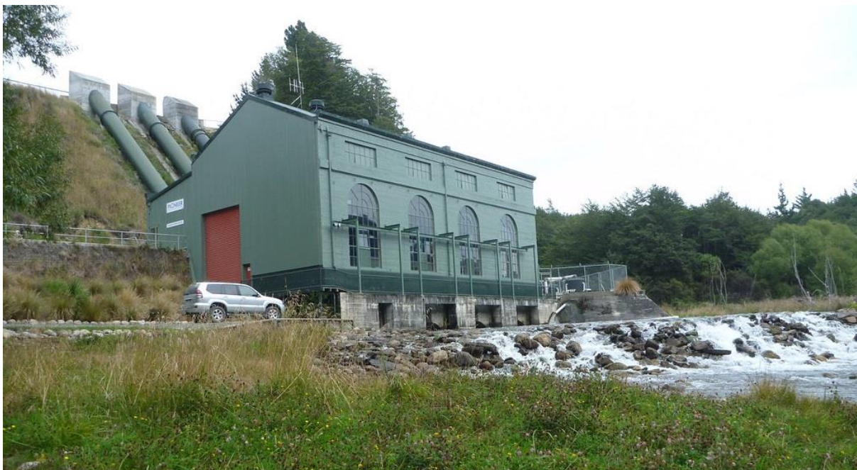
Figure 11: Monowai Power Station
