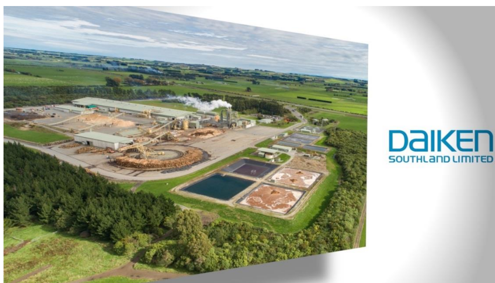
Figure 14: Aerial view of Daiken Southland site (Image by Daiken Southland Limited)
