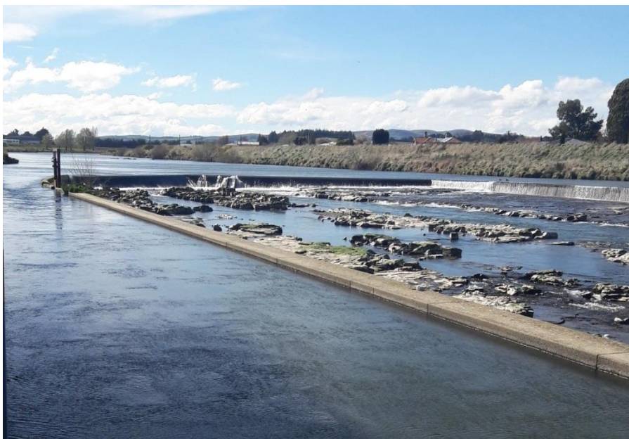
Figure 9: Upstream sampling site, Alliance Group Mataura Plant
