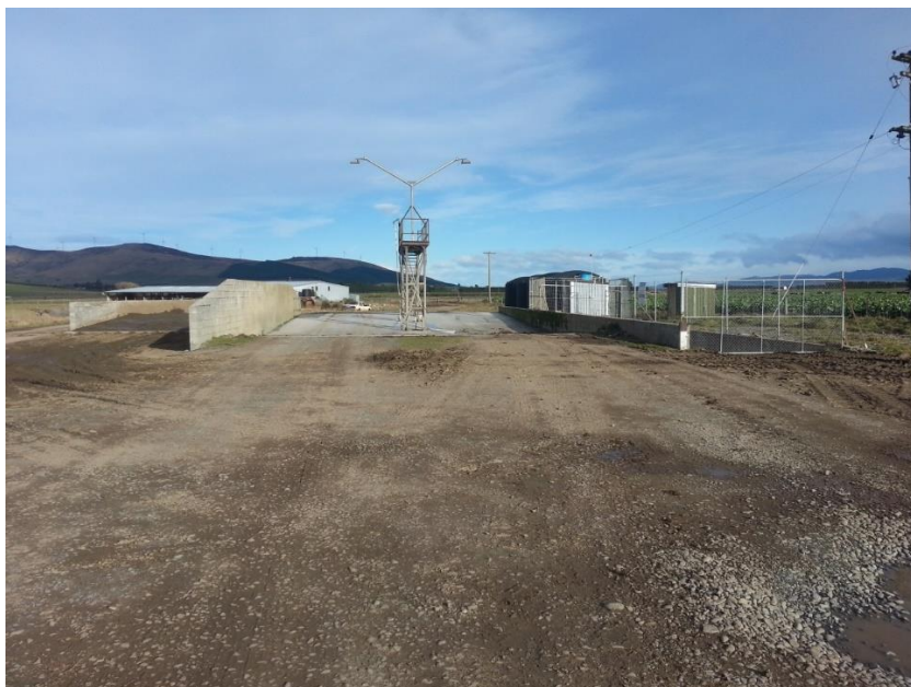
Figure 24: An example of a truck wash facility
