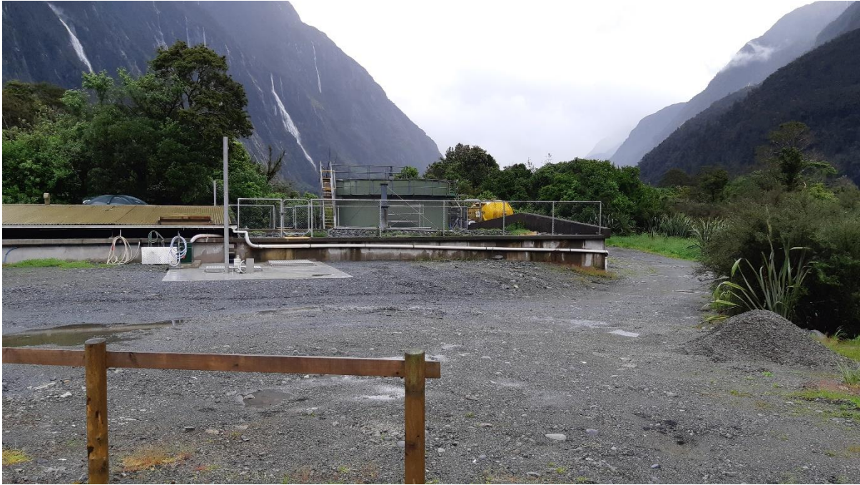
Figure 21: Milford Sound wastewater treatment plant
