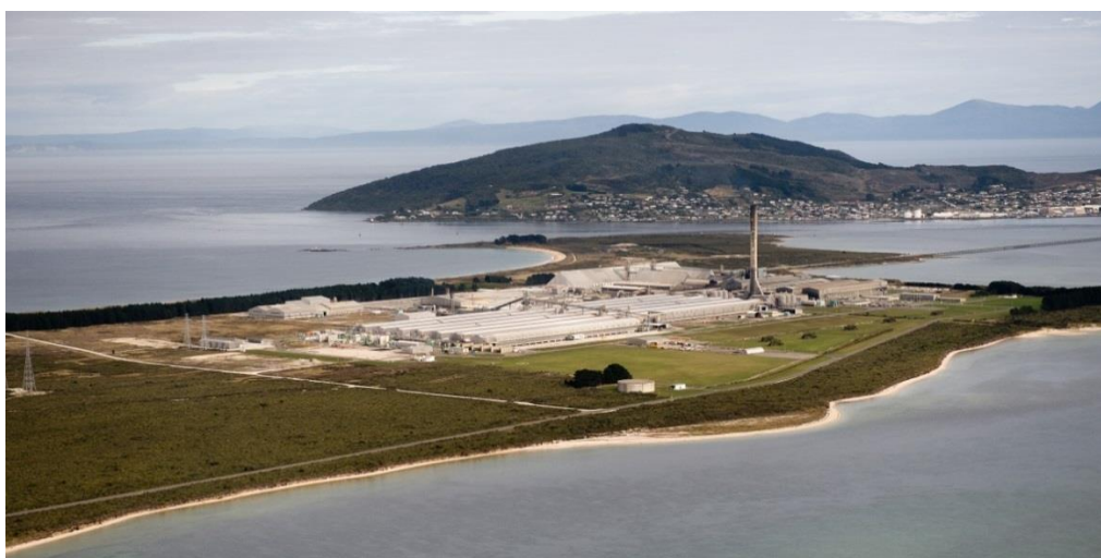
Figure 11: Aerial view of NZAS site. (Image by NZAS)
