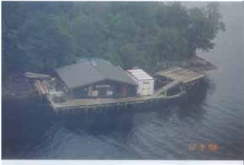
Figure 16 – A structure in Blanket Bay
