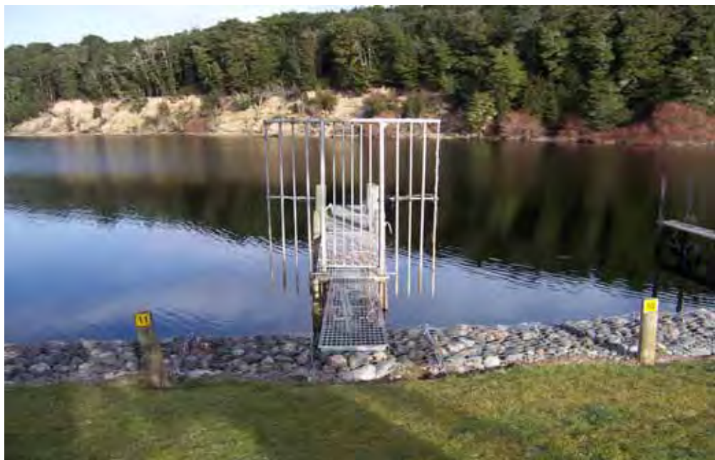
Figure 29 – Locked gate on structure at Manapouri
