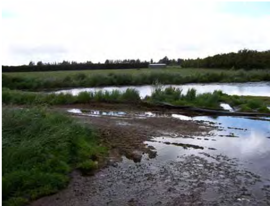
Figure 79 – Overflowing wintering pad pond
