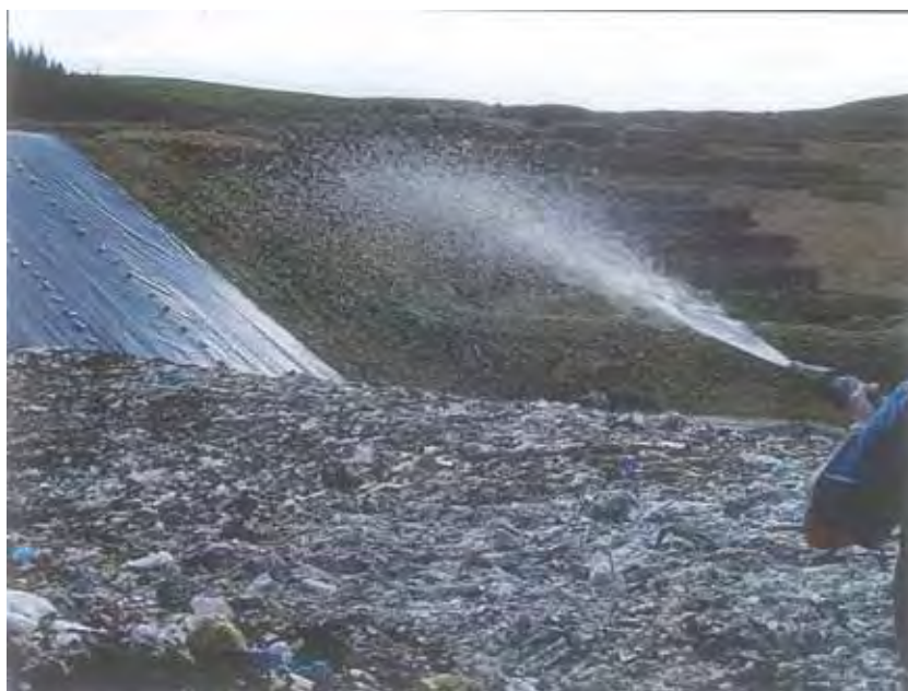
Figure 66 - Contractor applying the alternative daily cover to the landfill waste
