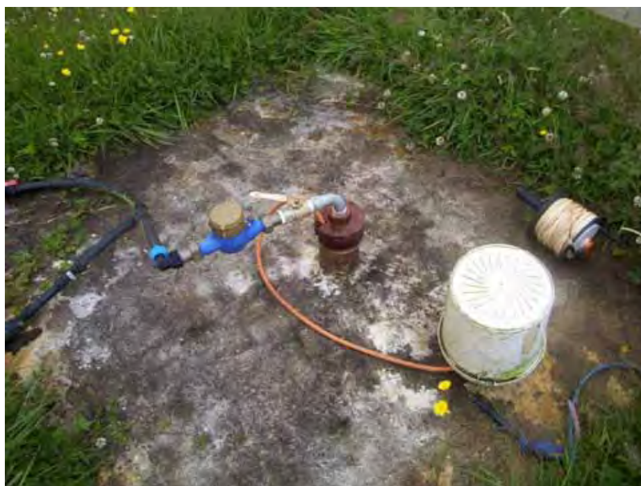
Figure 8 – An ideal bore set up: sealed to prevent contamination and fitted with a flow meter
