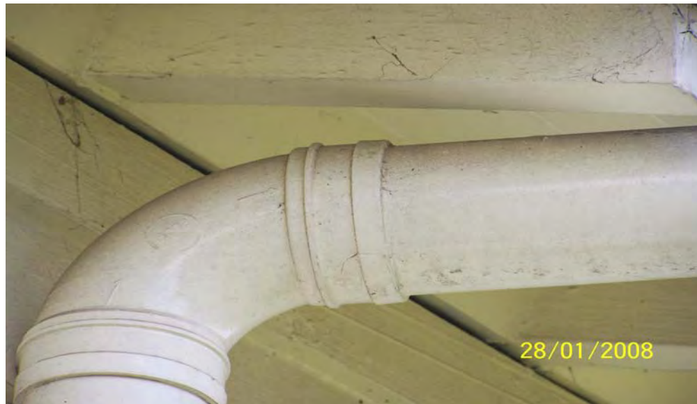
Figure 42 - Coal dust on neighbouring property
