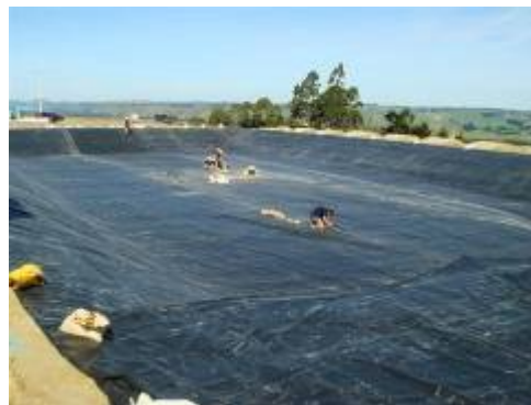
Figure 12 – Membrane pond liner
