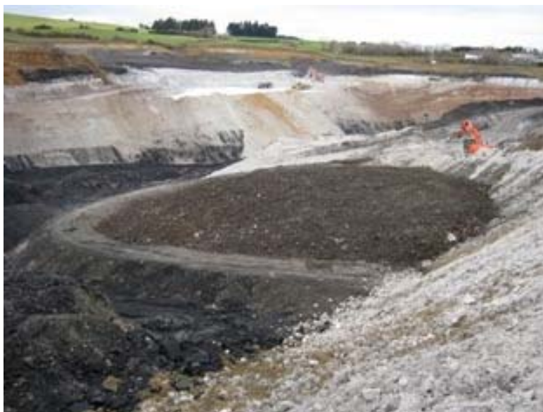
Figure 64 - Capping of relocated Nightcaps landfill – photograph supplied by Takitimu Coal Limited
