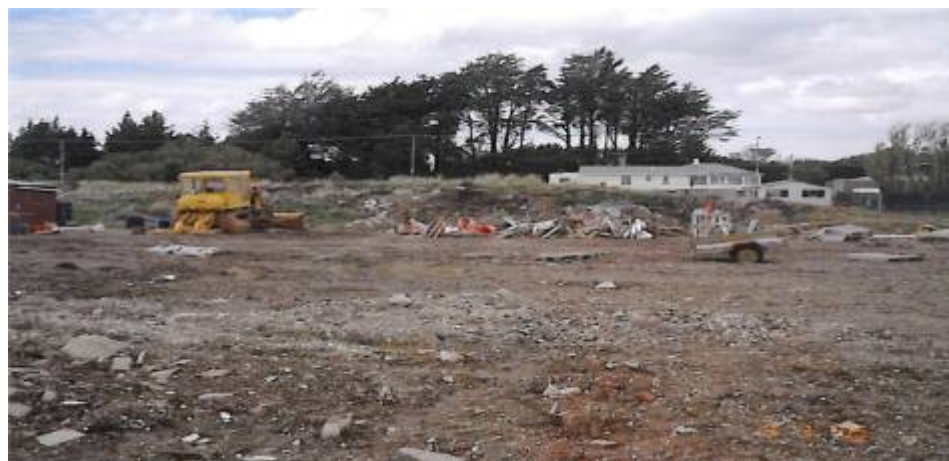
Figure 62 - A good management practise of stockpiling unacceptable cleanfill materials (metals, treated timbers) for future transfer to a recycling or lawful site.
