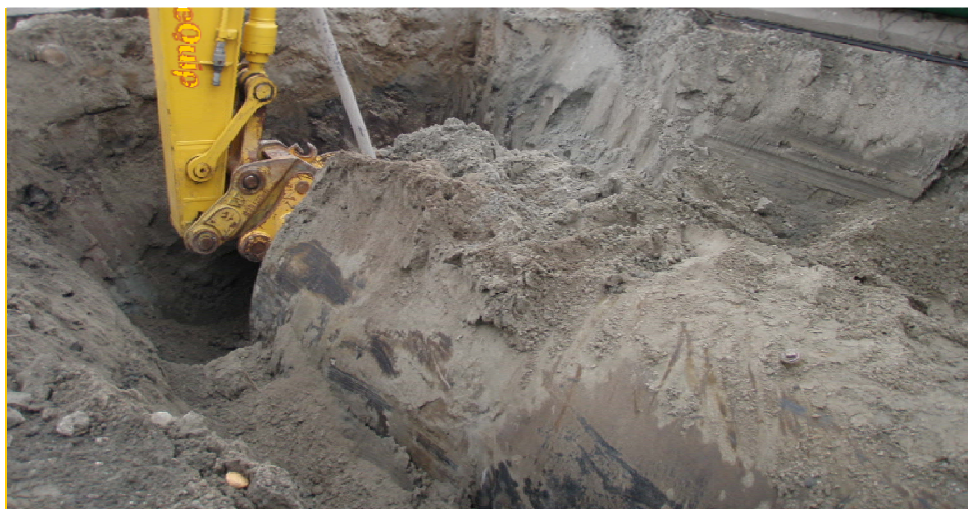
Figure 2 -The removal of an underground storage tank
