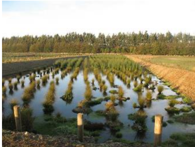
Figure 56 - One of the Matura oxidation pond wetland cells
