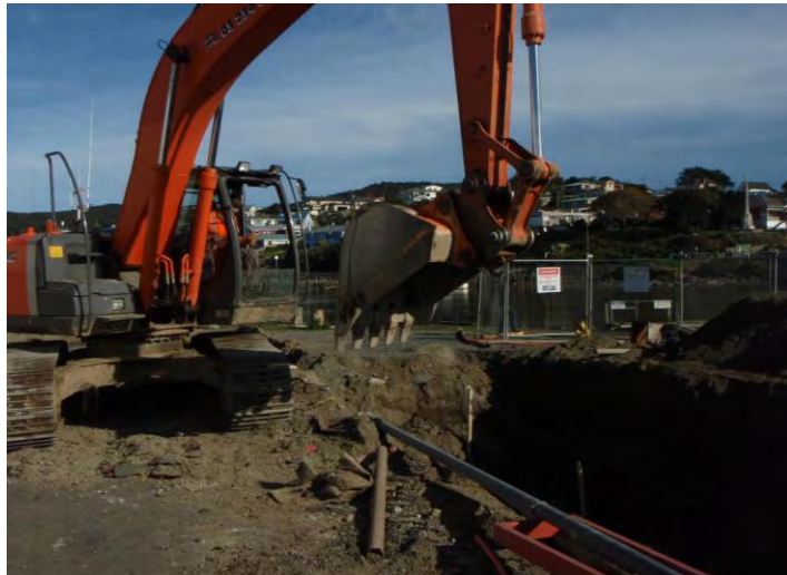
Figure 9 – Using excavator bucket to collect soil from pit for sampling.
