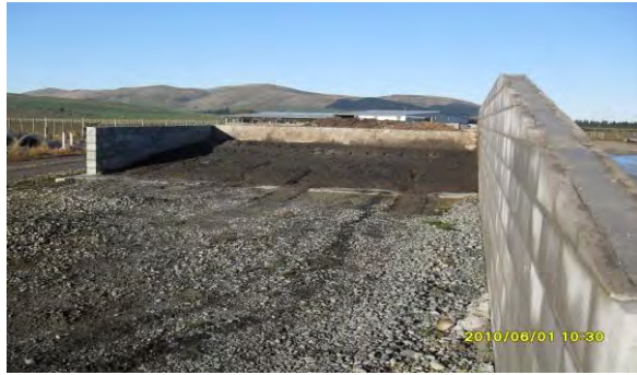
Figure 20 – Containment facility – sludges.
