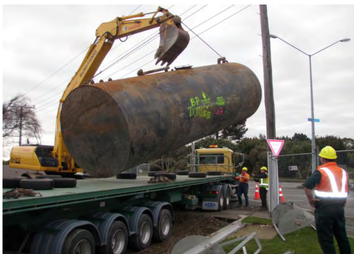
Figure 8 – Tank being loaded onto truck for assessment and recycling.
