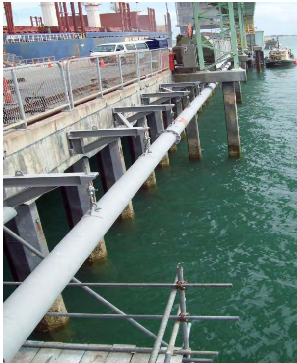
Figure 58 - After: HFO pipe line repositioned alongside the wharf.
