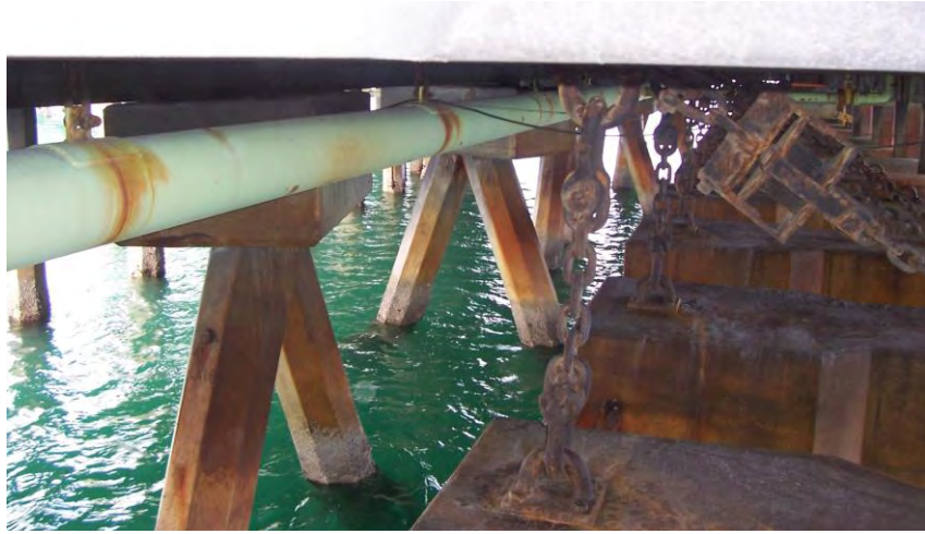
Figure 57 – Before - HFO pipeline running underneath the wharf.
