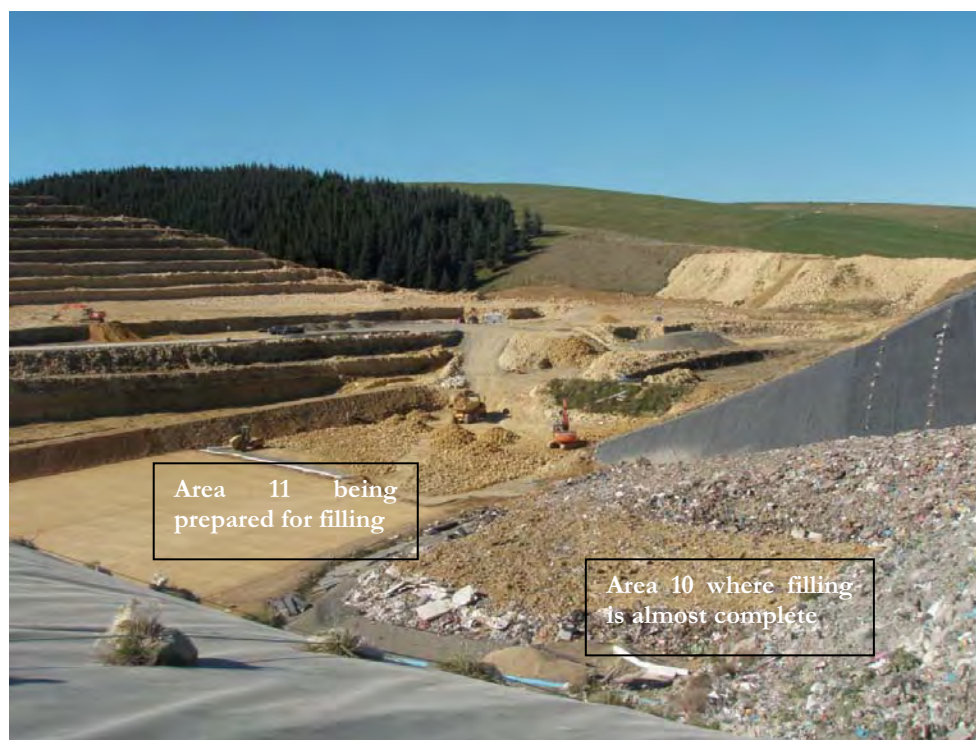
Figure 73 – View from edge of Area 10 towards Area 11, which was being prepared to accept waste.
