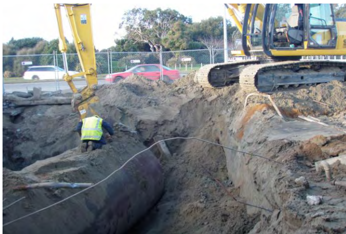
Figure 7 - Excavator at work removing tank from pit.
