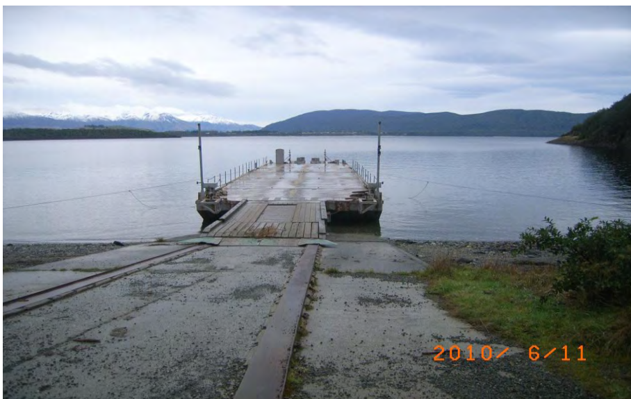
Figure 18 - Concrete ramp with a large barge.
