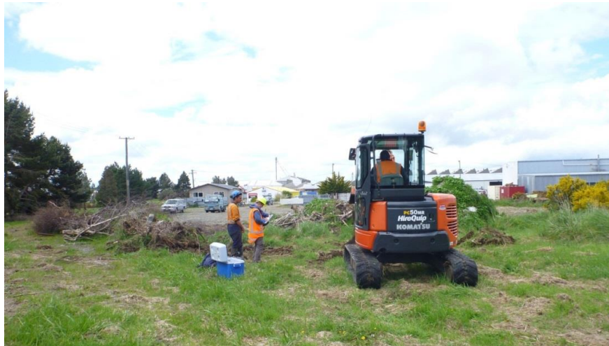
Figure 18 - Site investigation, Tweed Street, west Invercargill.
