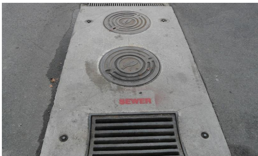
Figure 15 - Vehicle yard wastewater is treated and plumbed to sewer.
