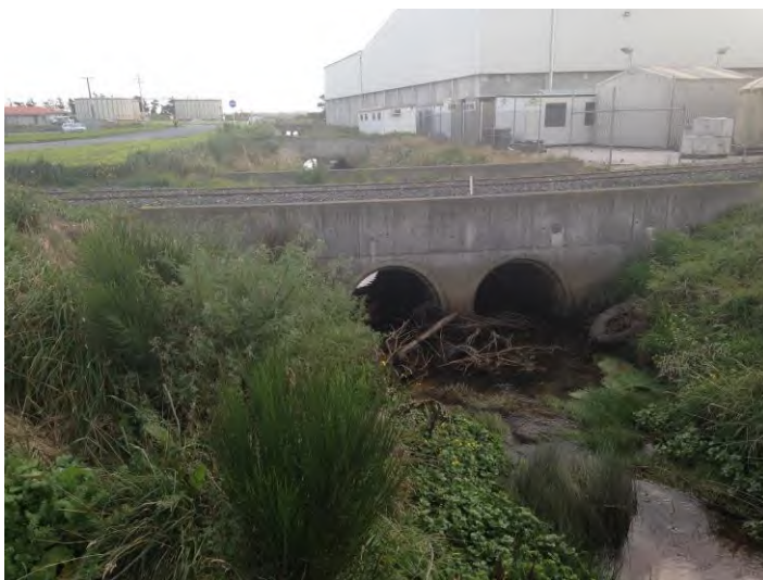
Clifton Channel near the Clifton Wastewater Treatment Plant
