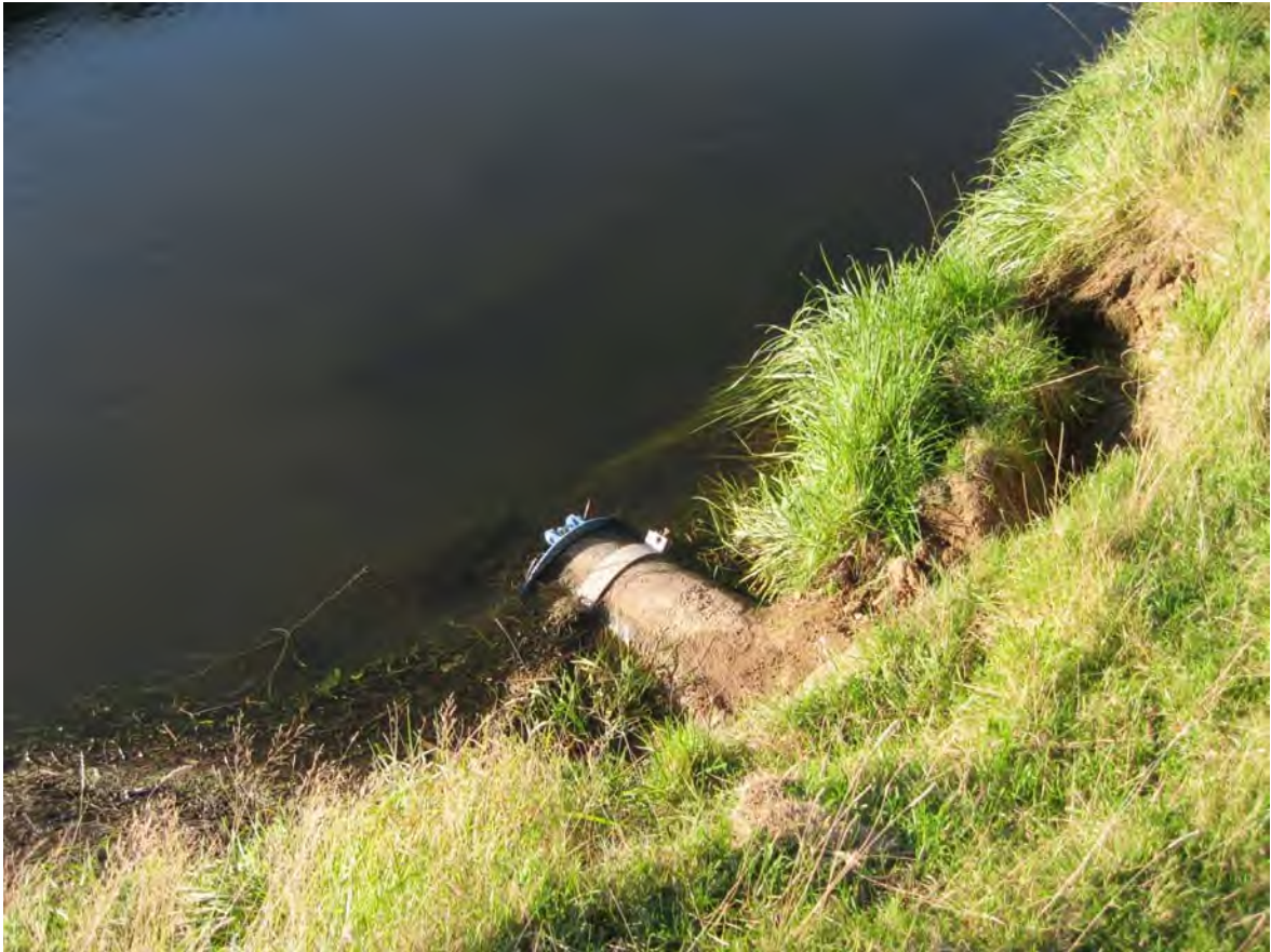
Figure 17 Stormwater drain entering Waikiwi Stream upstream of West Plains Road Bridge, Invercargill. View taken from true left, April 2016.
