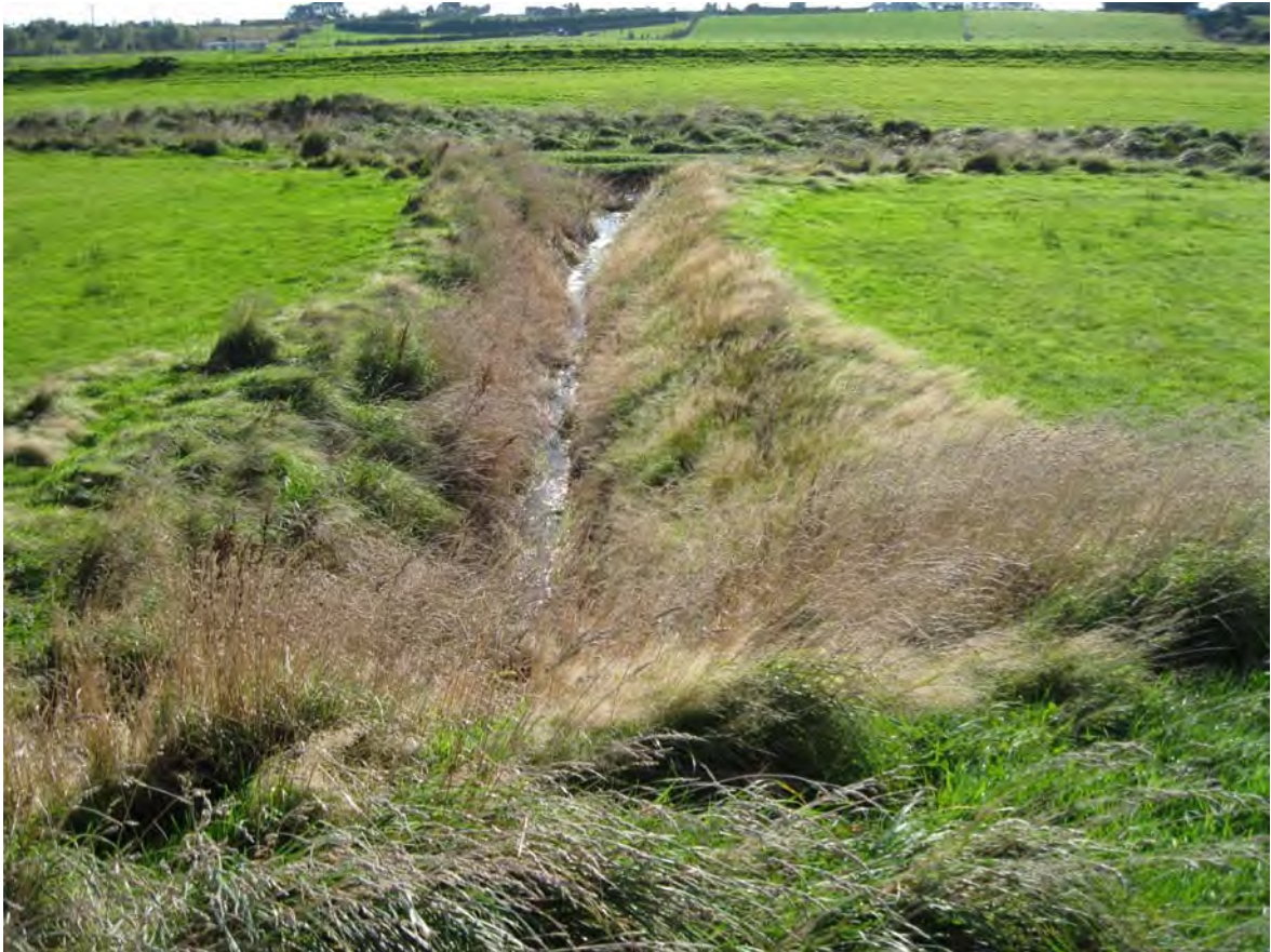
Figure 13 Downstream view of a stormwater drain that enters the Waihopai River near Racecourse Road, Invercargill, April 2016.
