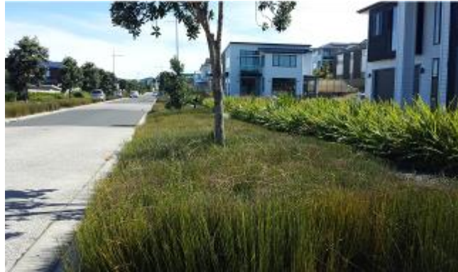
Figure 2 Rain gardens in road reserves, Long Bay, Auckland
